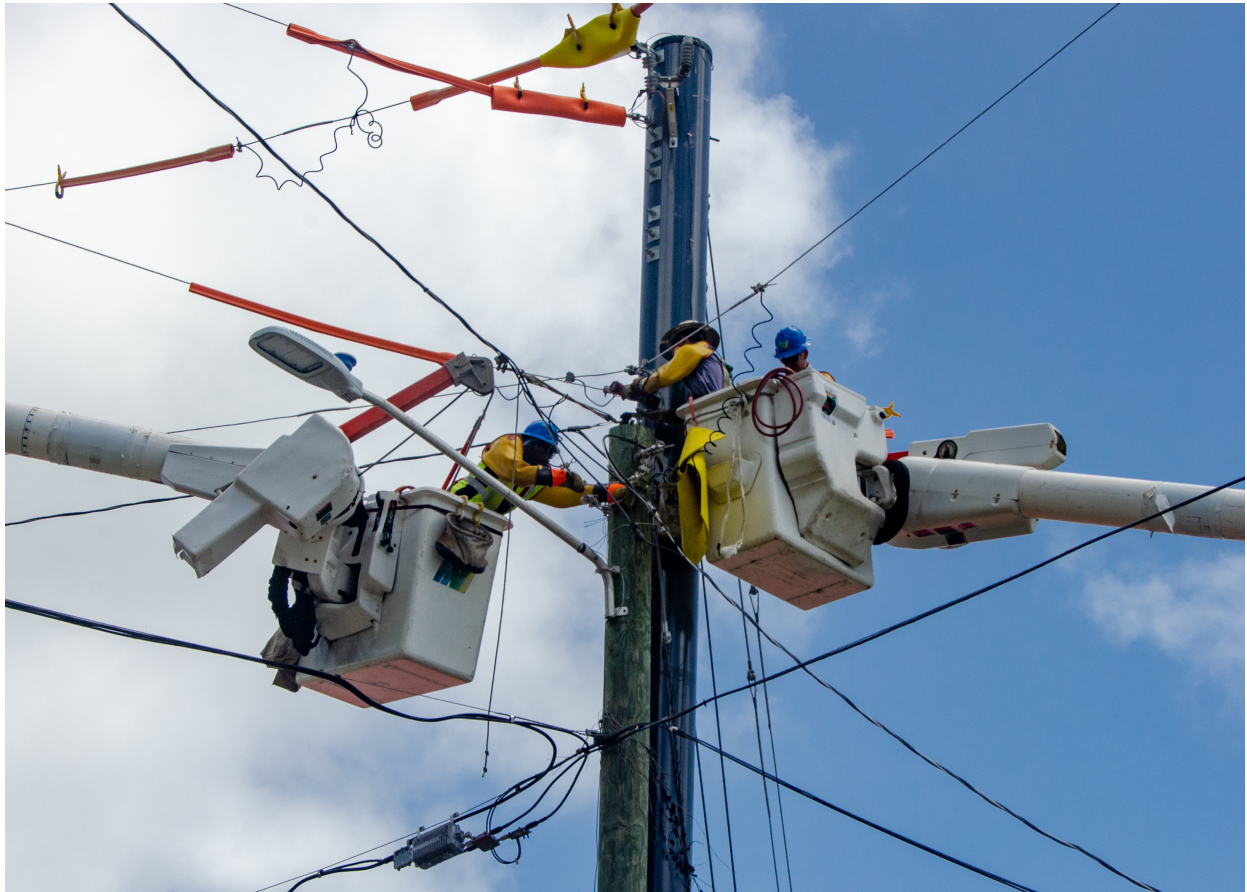
Haugland Virgin Islands line workers finish installation of a composite power pole in July 2021 in Upper Contant on St. Thomas. The Virgin Islands Water and Power Authority is leading operations to install 2,333 composite poles on the island. FEMA/Eric Adams
