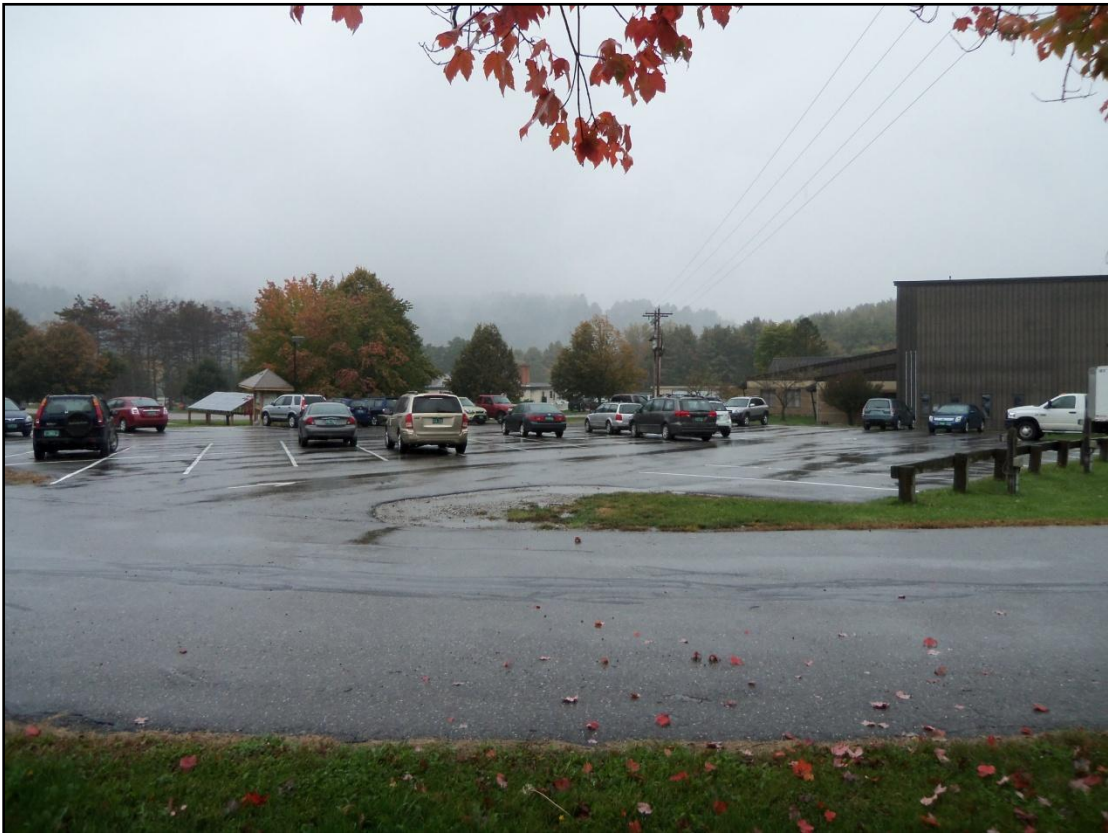
Site Photo 6: Looking west from behind ball field, to existing parking lot, to be used by new temporary facility
