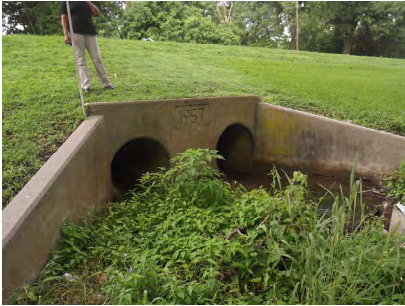
Figure 7: Existing Headwall at Lake Providence Outfall
