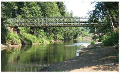
To provide a crossing of the Chehalis River after the three bridges were destroyed, the Washington State Department of Transportation (WSDOT) installed a temporary modular bridge (called a Bailey bridge) just upstream of the former Leudinghaus Road Bridge site, on loan to Lewis County. The Bailey bridge, pictured on site at left, had some important limitations. The temporary bridge was a one-lane bridge, and due to weight
