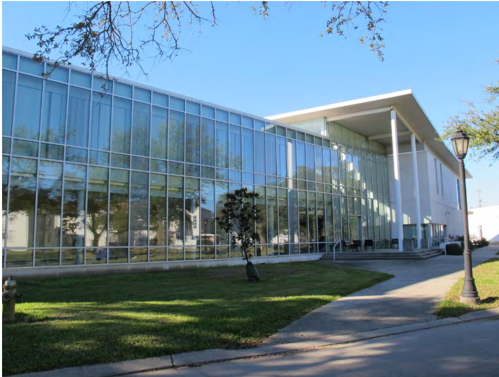
Figure 8. DUICEF Building, looking southwest. Photo taken by FEMA, January 2016.
