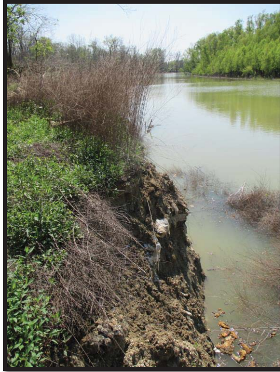
Figure 9. Revetment-1, facing southeast, displaying modern debris/trash deposit (03/15/2017).
