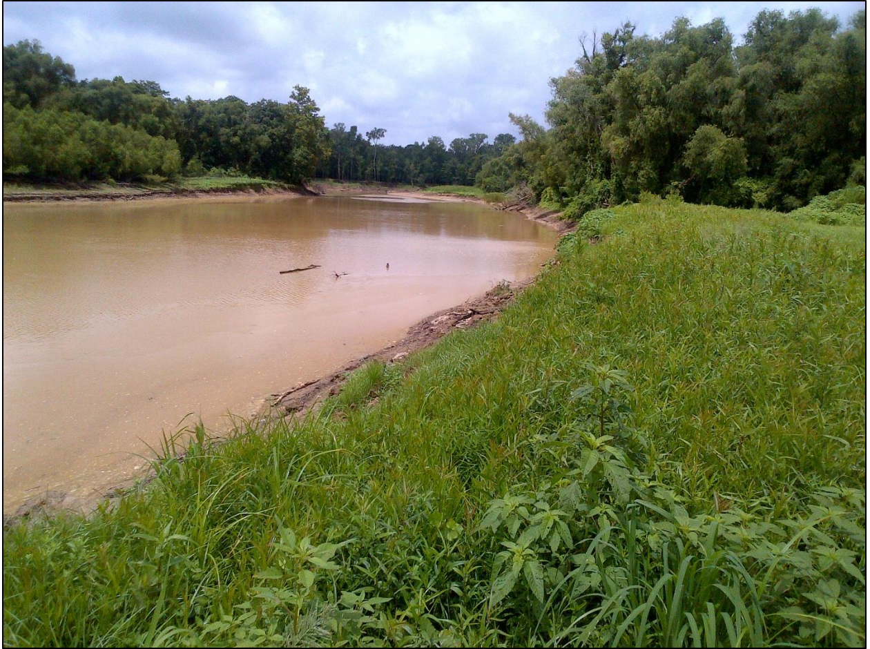
Photo 5 View from east bank of Bayou Sara, looking west/upstream (July 28, 2018).
