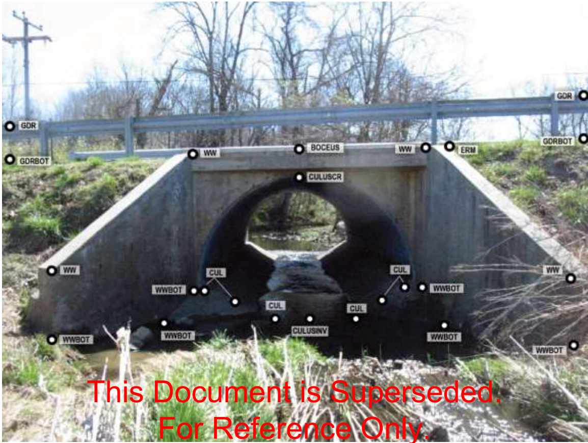
Figure 3: Typical Culvert Photograph: Sanderson Creek SAN-0880 (Displays Survey Code Locations)
