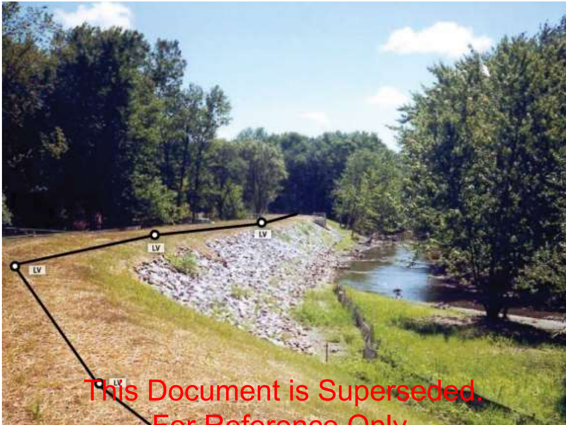
Figure 6: Typical Levee (Displays Survey Code Locations)
