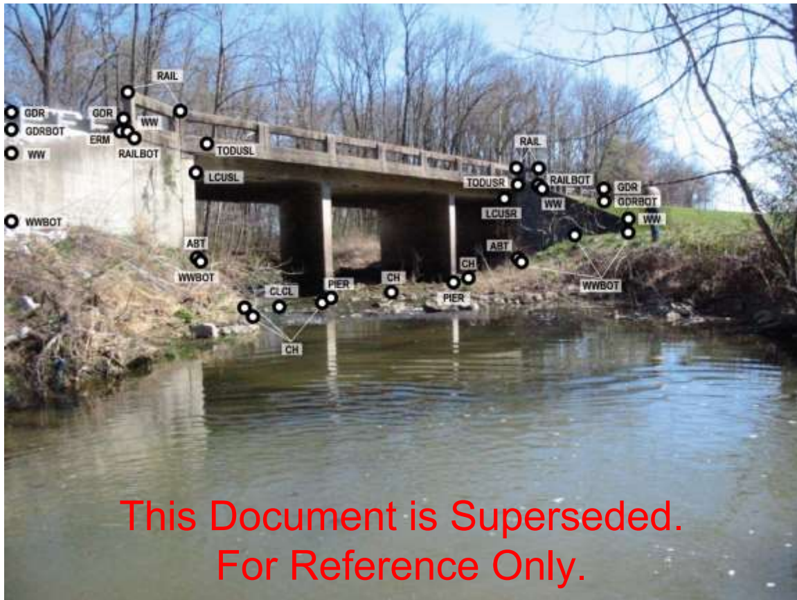
Figure 2: Typical Bridge Photograph: White Creek WHI-1800 (Displays Survey Code Locations)
