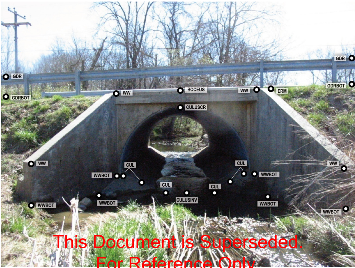
Figure 6: Typical Culvert Photograph (Displays Survey Code Locations)
