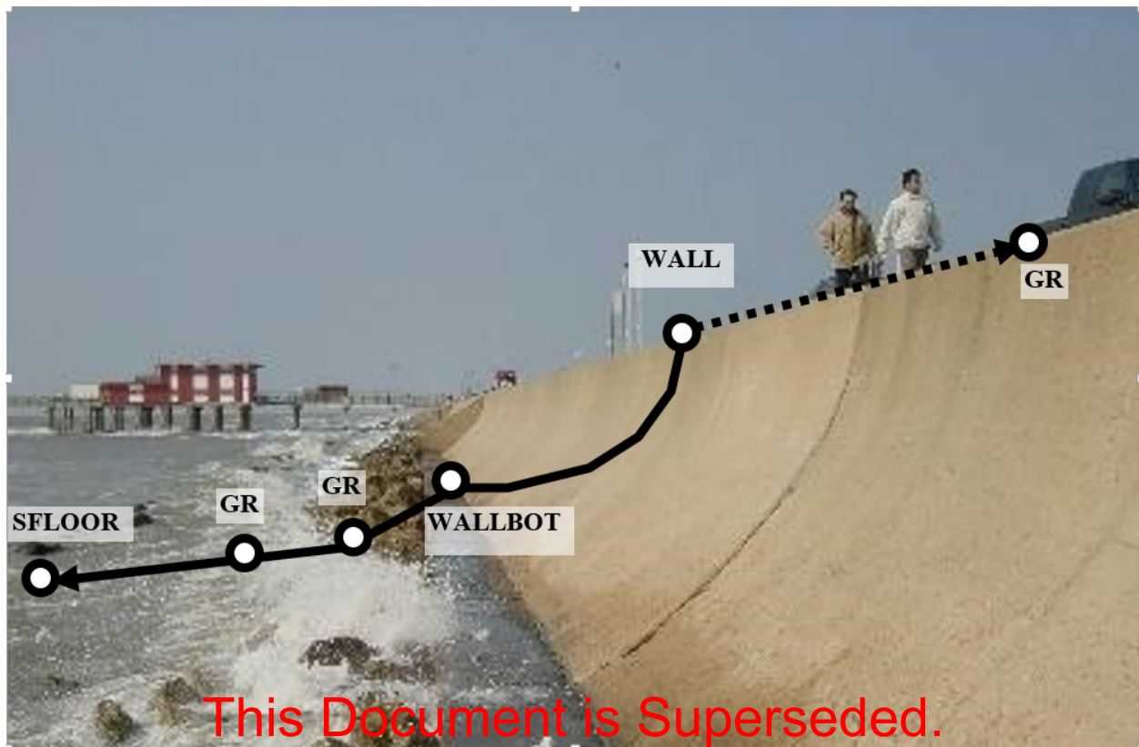
Figure 14: Typical Coastal Structure Photograph (Displays Survey Code Locations)
