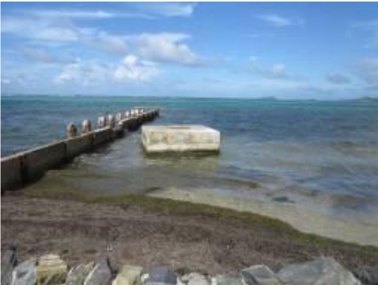
Photograph 2. Photograph of MH 0436, between Colony Cove and Mill Harbor. The photograph illustrates the erosion into the seagrass bed. (Photograph courtesy of Bioimpact, Inc.).
