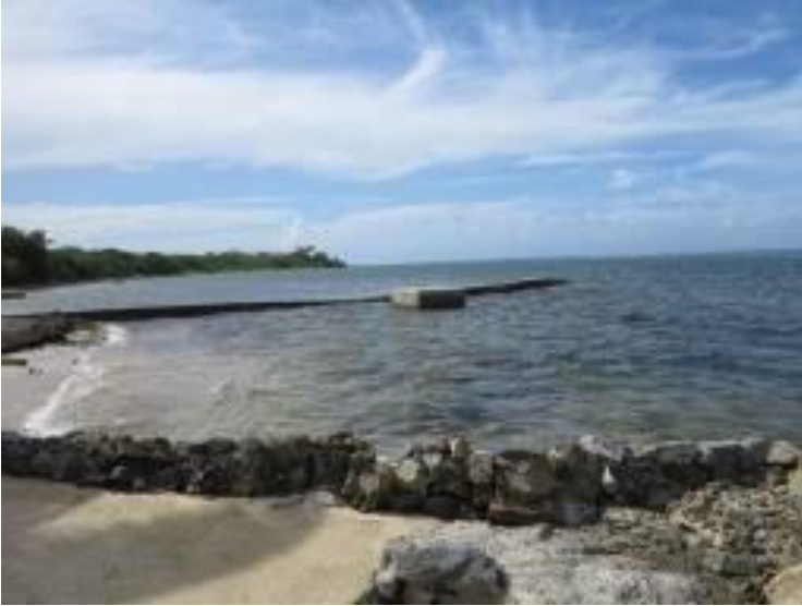
Photograph 3. This photograph shows MH 0435 off of Mill Harbour adjacent to a groin which was constructed to maintain the sand on Mill Harbour's Beach. (Photograph courtesy of Bioimpact, Inc.).
