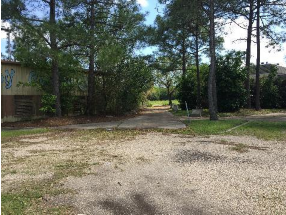
Photo 13 – View of the two main buildings on the former Brechtel Golf Course site.
