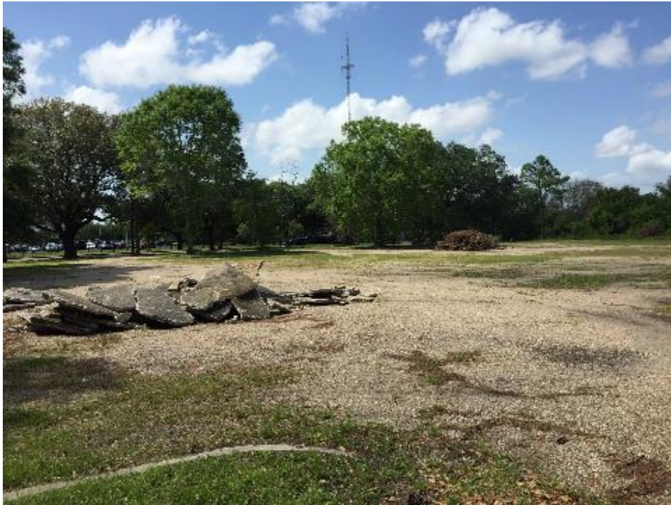
Photo 14- View of concrete pile onf the former Brechtel Golf Course site.
