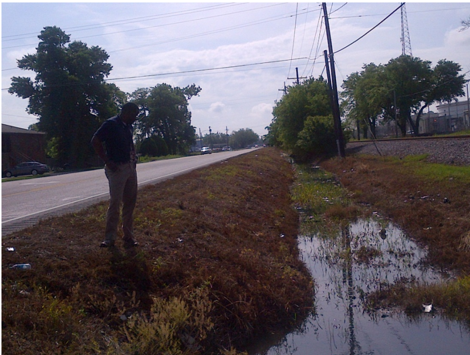
Figure 5: Plaza Drive Pump Station – Discharge ditch from Plaza Drive pump station
