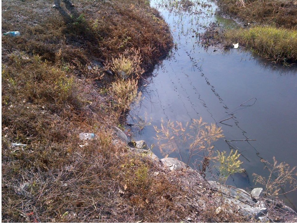
Figure 4: Earthen discharge ditch on East St. Bernard Hwy across from Plaza Drive pump station
