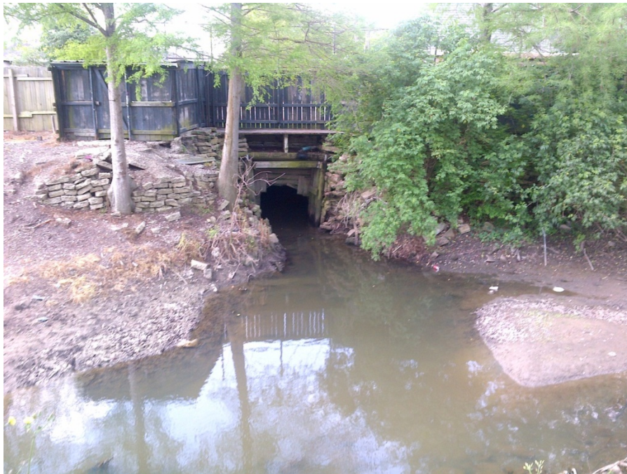
Figure 12: Existing culvert emptying into the 20 Arpent Canal
