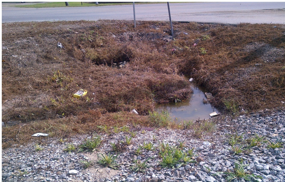
Figure 7: Plaza Drive Canal Culvert #2 proposed to be replaced
