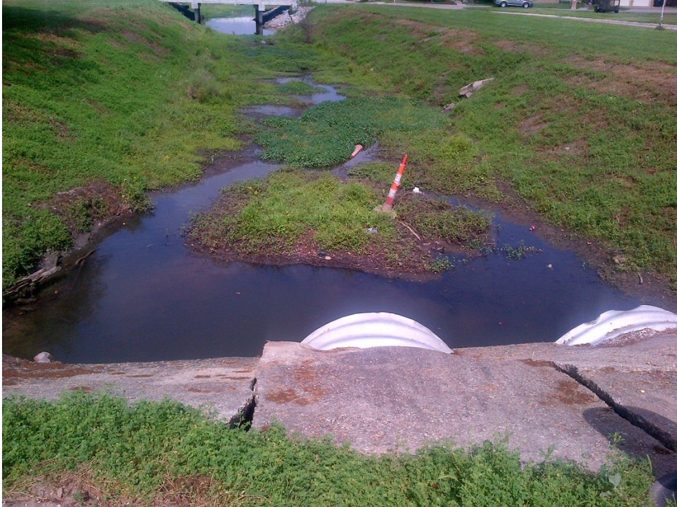
Figure 15: 20 Arpent Canal looking downstream to chape canal
