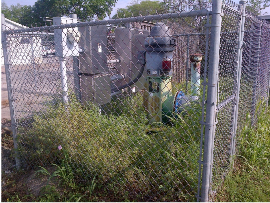
Figure 2: Existing Plaza Drive Pump Station to be replaced
