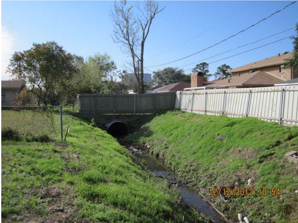
Photograph 1. Culvert Installed in Channel
