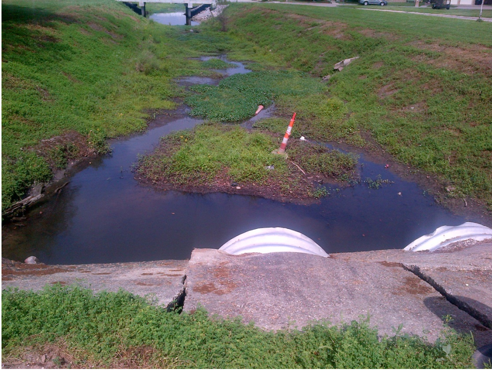
Figure 15: 20 Arpent Canal looking downstream to chape canal
