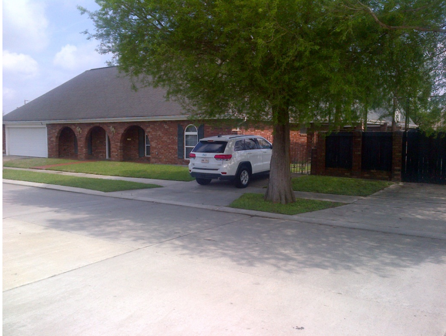
Figure 13: 1201 Missouri Street –Proposed House to be demolished
