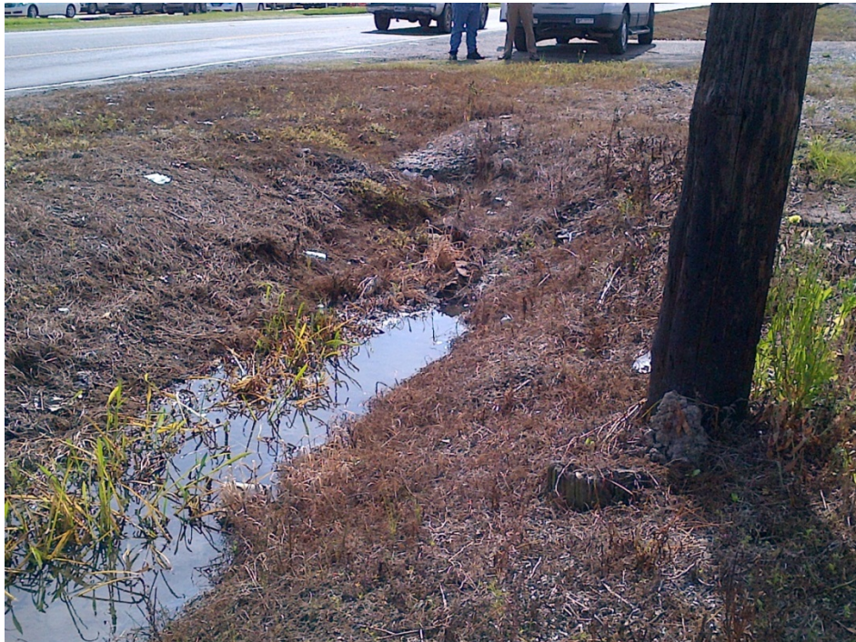
Figure 6: Plaza Drive Canal Culvert #1 proposed to be replaced
