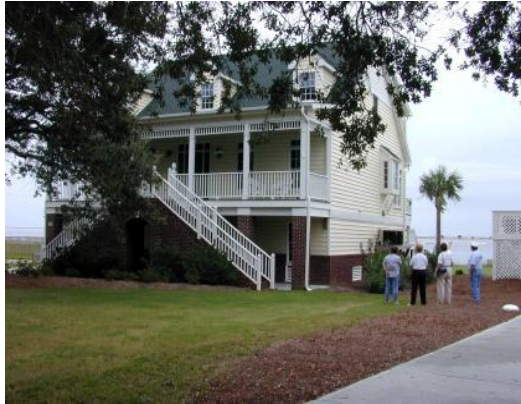
Mitigation: Elevating a home by the river
