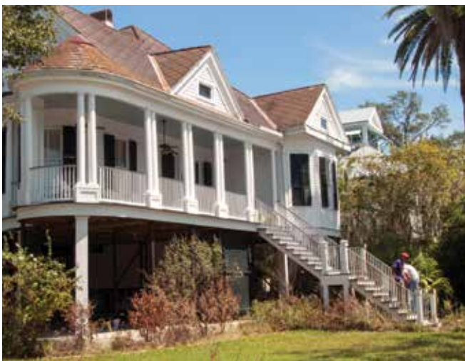
This older home in Mandeville, Louisiana, sustained only minor flood damage during Hurricane Isaac because it had been elevated after Hurricane Katrina
