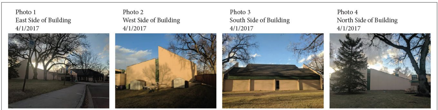
Figure 3. Photos showing the structure to be retrofitted. Photos include all sides of the building from different cardinal directions.
