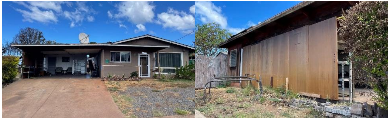
Figure 20. House with attached carport in Lahaina, with carport side support wall constructed or repaired using leftover door panels.
