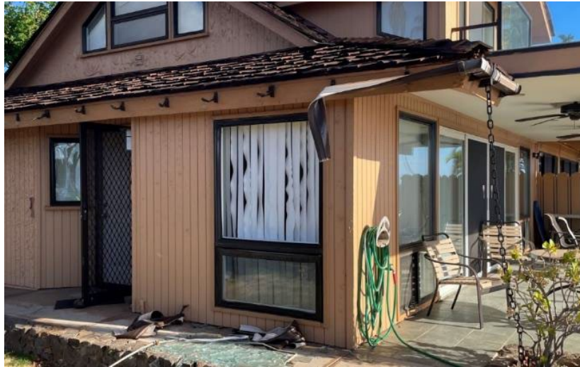
Figure 10. Melted vinyl gutters and melted window frame with lost glass pane on a residential building in Lahaina.
