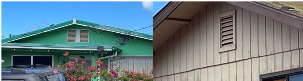
Figure 13. Examples of gable end louvred vents.
