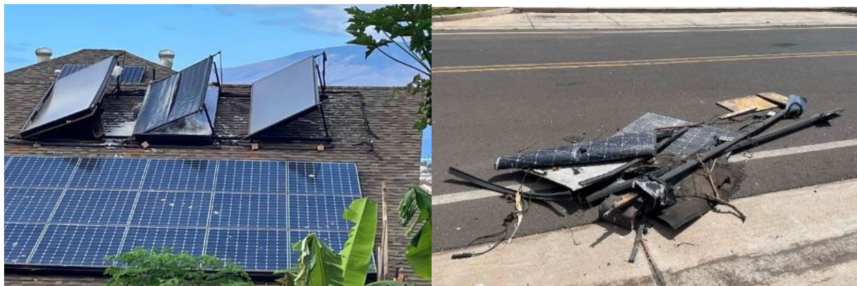
Figure 11. Damaged solar water heaters observed on a residential building in Lahaina (left). PV panels found on the ground along a street lined with single-family residential buildings in Lahaina (right).
