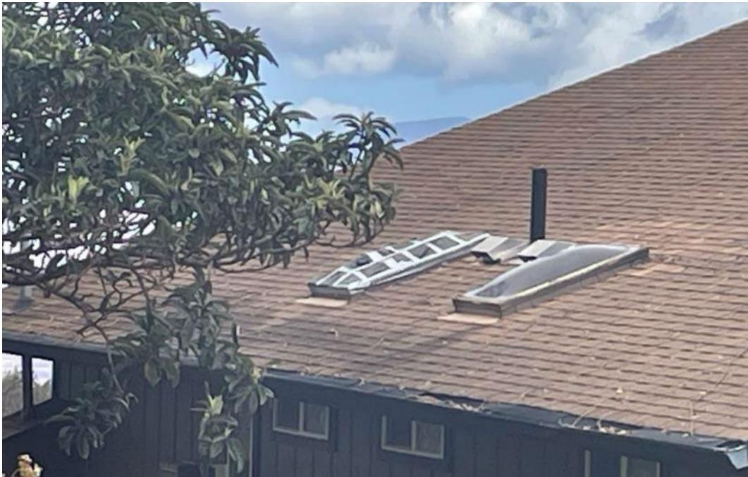
Figure 18. Older plastic skylight on a residential building in Kula damaged by wildfire.
