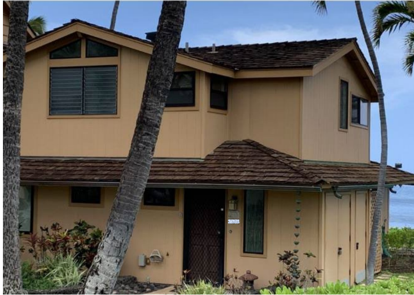
Figure 9. Wood shake roof on a residential building in Lahaina, showing evidence of some surface shakes charred by fire.
