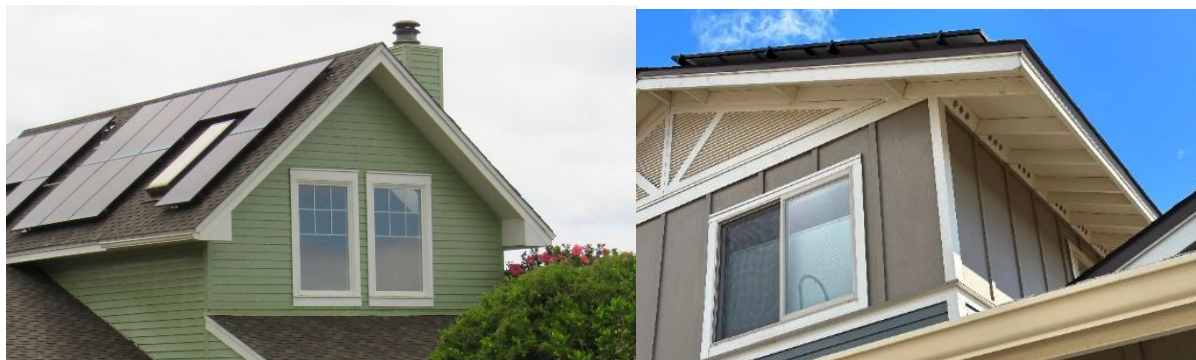
Figure 12. Typical closed Soffit on Maui residential building (left). Open soffits with small “birdhole” vents on residential units in Lahaina created by an extension of roof framing (right).
