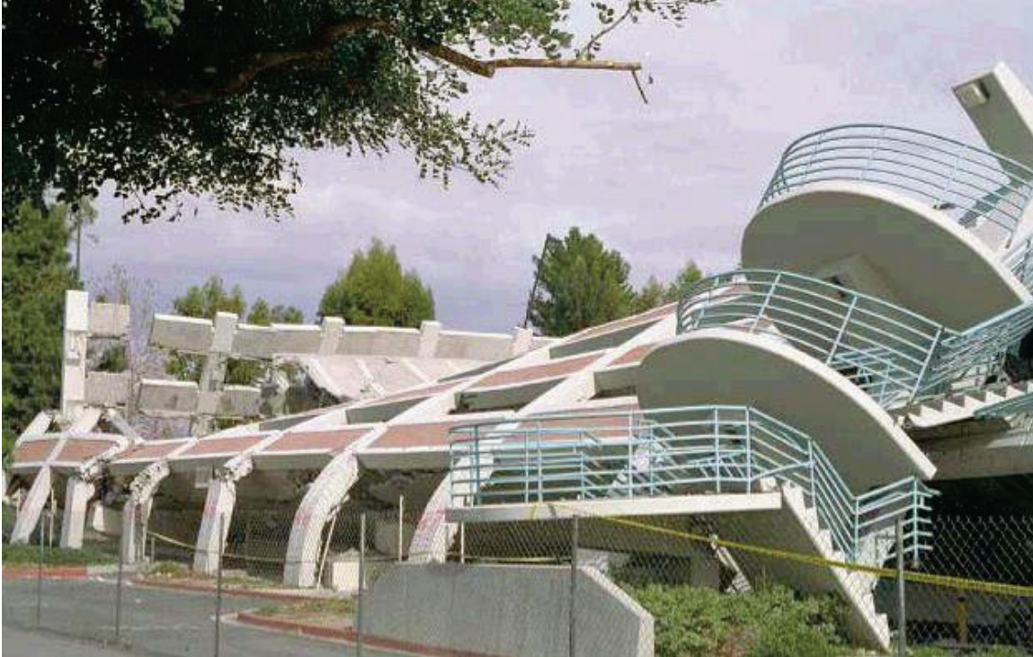
Figure 3-36 Parking garage damage at Northridge CSU in the 1994 Northridge Earthquake (Exponent/Shusto).
