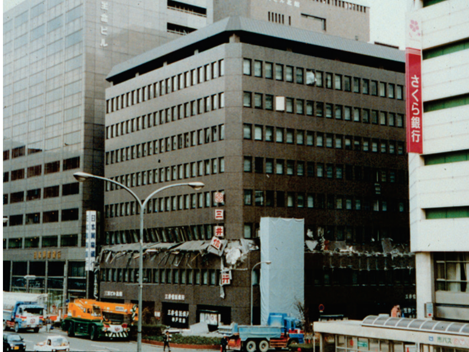
Figure 3-14 Third story collapse of 10-story office building in 1995 Kobe Earthquake in Japan (Source: Exponent/Osteraas).
