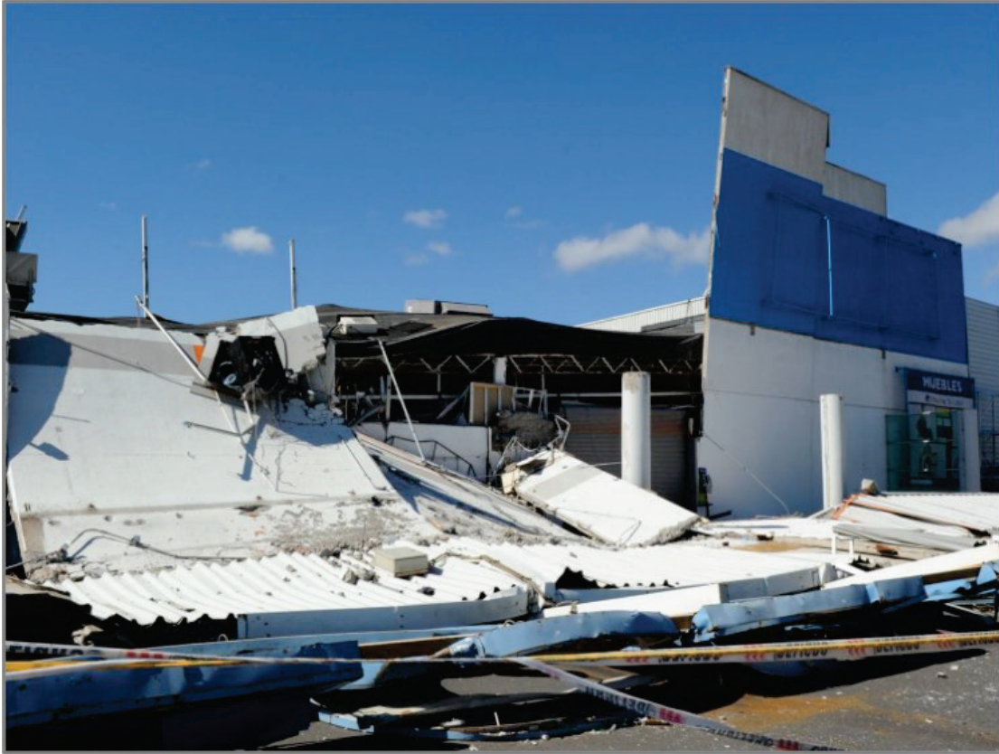
Figure 3-31 Collapse of tilt-up walls in the 2010 Maule, Chile Earthquake (ATC-20 training slides).
