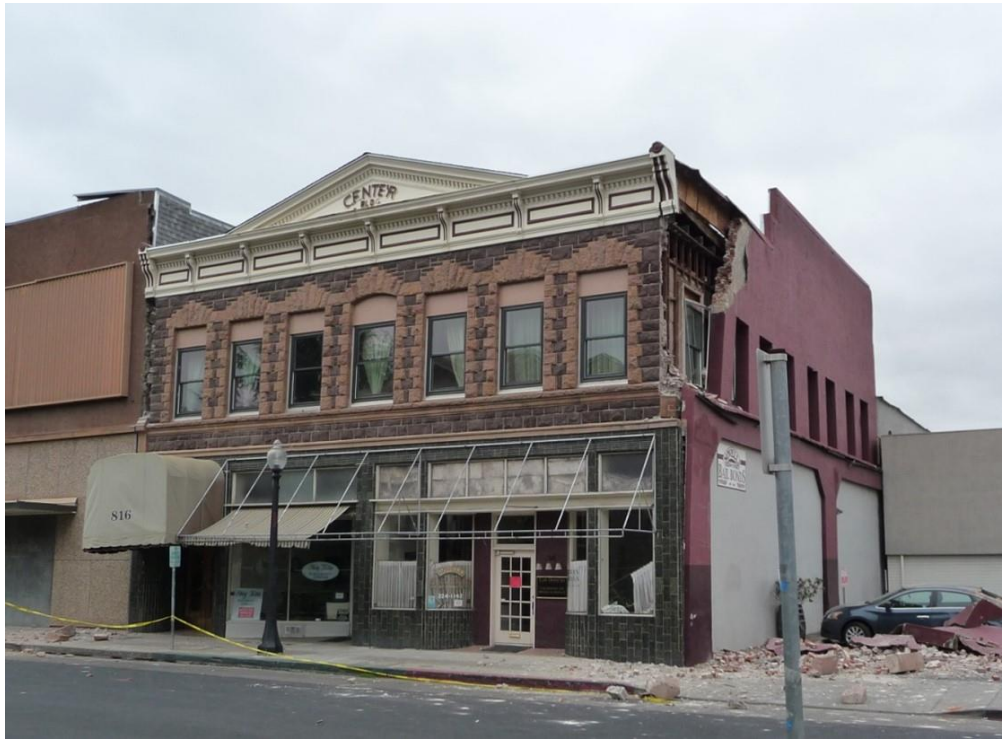
Figure 2-4 Failure of URM south wall of URM building posted UNSAFE (FEMA P-1024 Figure 4-49, photo by Marko Schotanus).
