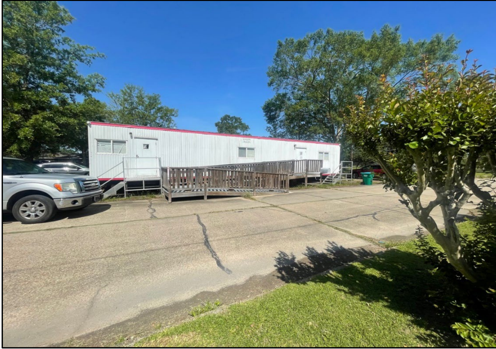
Figure 2 – Existing DSHA Administrative Building located at original facility location at 600 Eugene Street.
