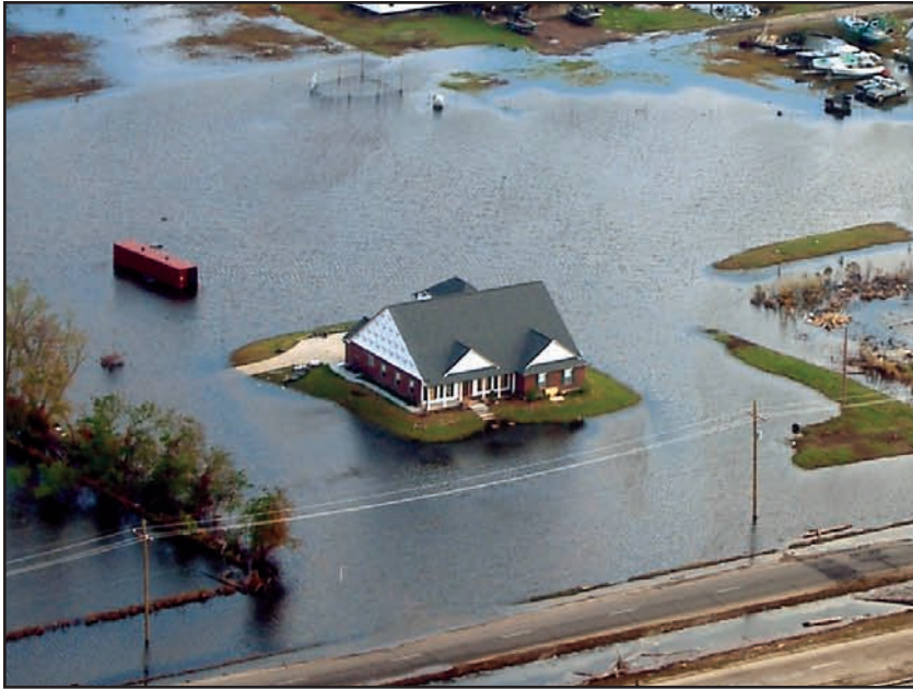
Figure 6-4. PLAQUEMINES PARISH, LOUISIANA: Home that had been elevated on fill, during the aftermath of Hurricane Katrina. (Source: FEMA 549)
