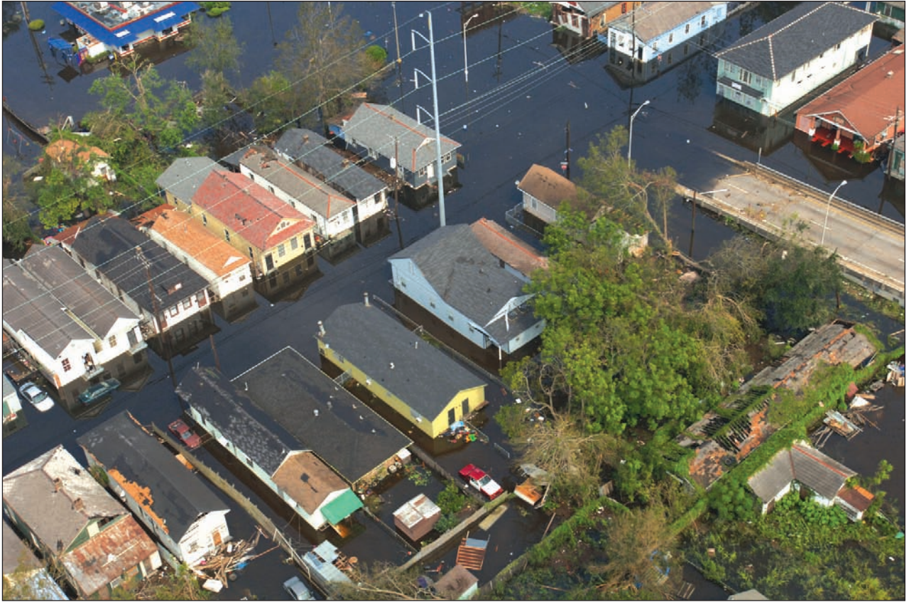
Figure 2-27. NEW ORLEANS, LOUISIANA: Neighborhood with homes flooded and cars covered. In the background is a breached levee with water entering the area. (Source: FEMA 549)
