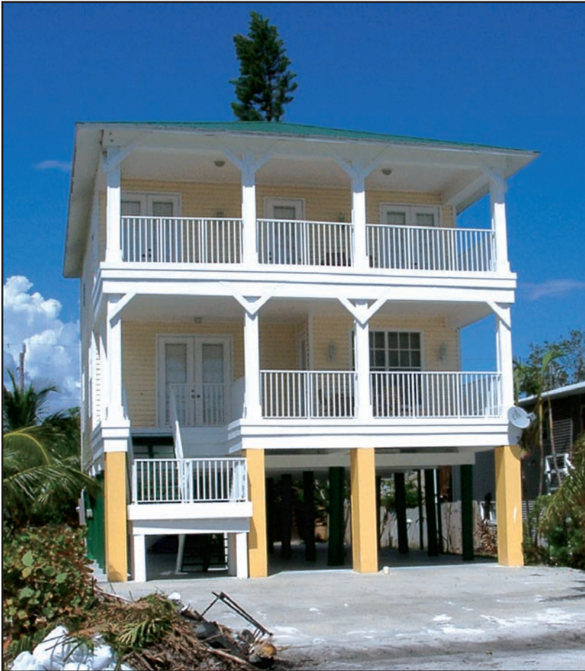
Figure 6-9. FORT MYERS BEACH, FLORIDA: Newly constructed house elevated on an open foundation sustained no storm surge damage when surges several feet deep impacted this site in 2004. (Source: FEMA 488)
