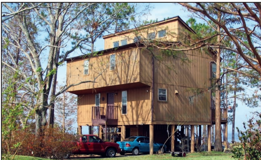
Figure 5-11. BIG LAGOON, FLORIDA: This house was elevated on piles, preventing major flood damage. (Source: FEMA 489)
