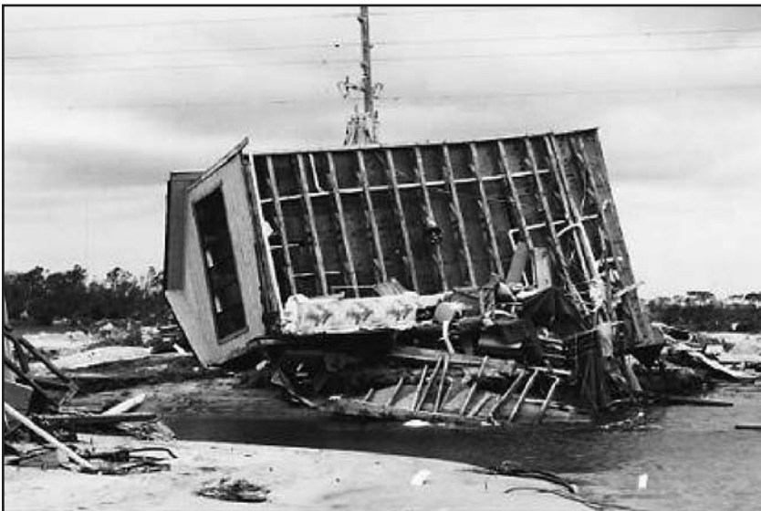
Figure 5-2. NORTH CAROLINA, HURRICANE FRAN (1996): Load path failure in connections between home and its foundation. (Source: FEMA 55)
