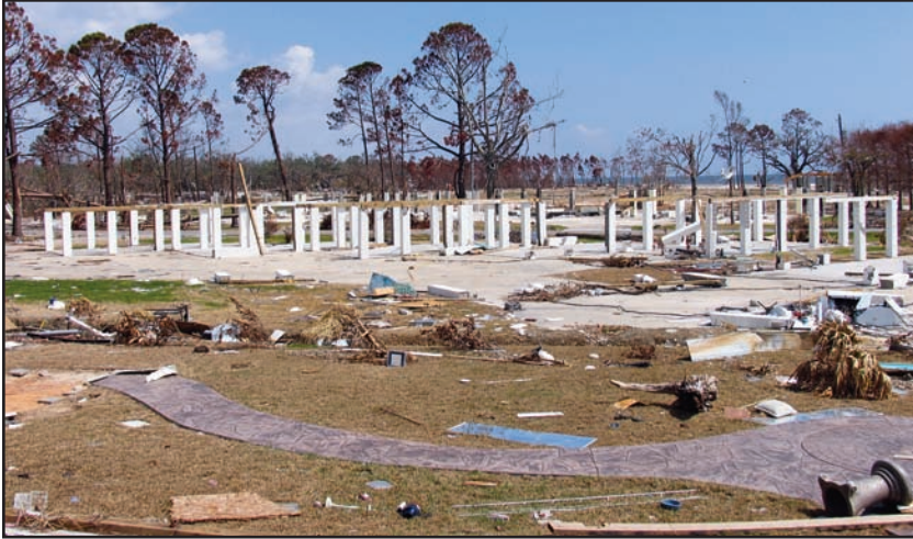
Figure 6-12. LONG BEACH, MISSISSIPPI: Structure removed from its foundation when waves exceeded the foundation height and connections between the elevated building and its foundation failed. The building was located within a mapped V Zone. (Source: FEMA 549)
