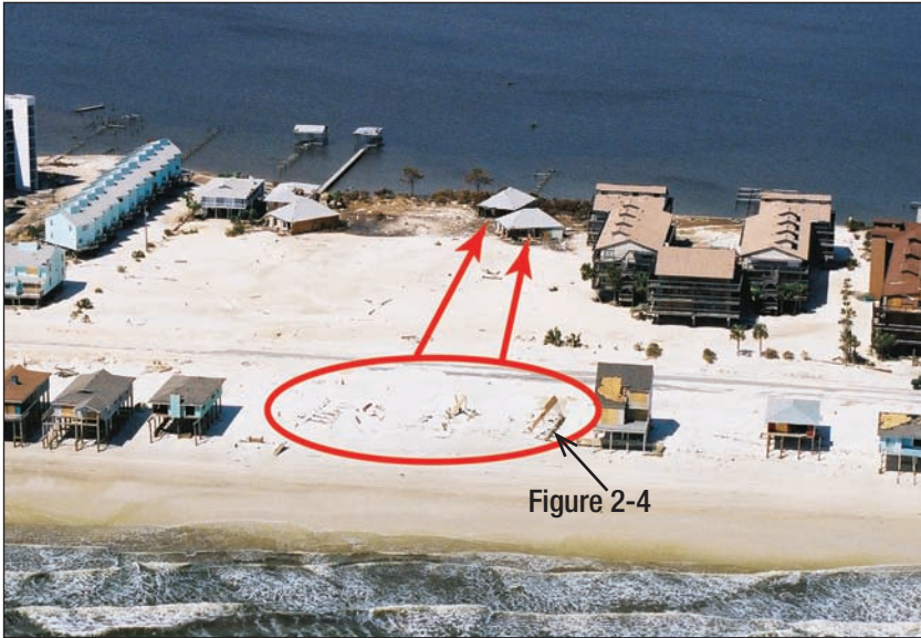
Figures 2-3 and 2-4. GULF SHORES, WEST BEACH, ALABAMA: Insufficient pile embedment contributed to the displacement of houses. (Source: FEMA 489)
