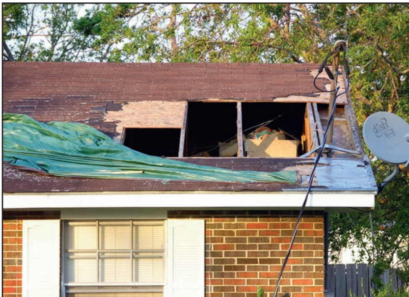
Figure 7-4. Loss of roof sheathing due to inadequate fastening between roof sheathing and framing. (Source: FEMA 549)
