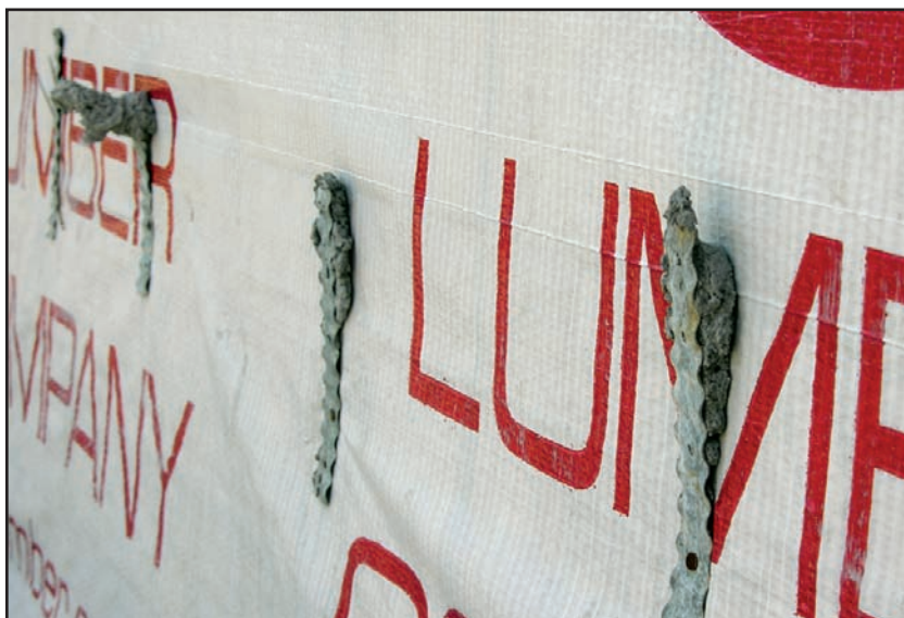
Figure 9-11. WAVELAND, MISSISSIPPI: House with collapsed brick veneer as a result of insufficient wall ties. (Source: FEMA 549)
