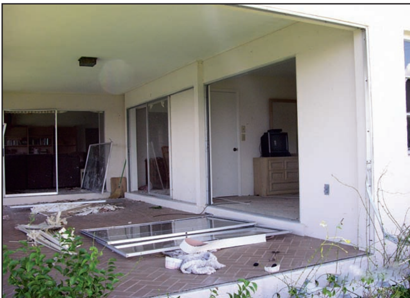
Figure 10-7. PUNTA GORDA ISLES, FLORIDA: Anchorage failure in sliding glass door failure. (Source: FEMA 488)
