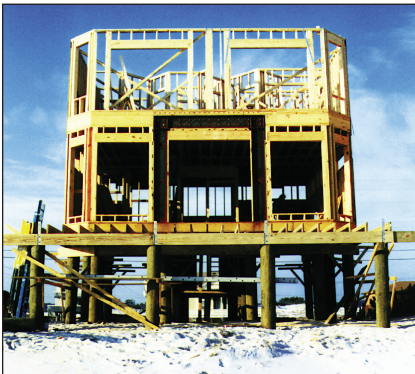
Figure 7-15. Residential use of a moment resistant frame. (Source: FEMA 55)
