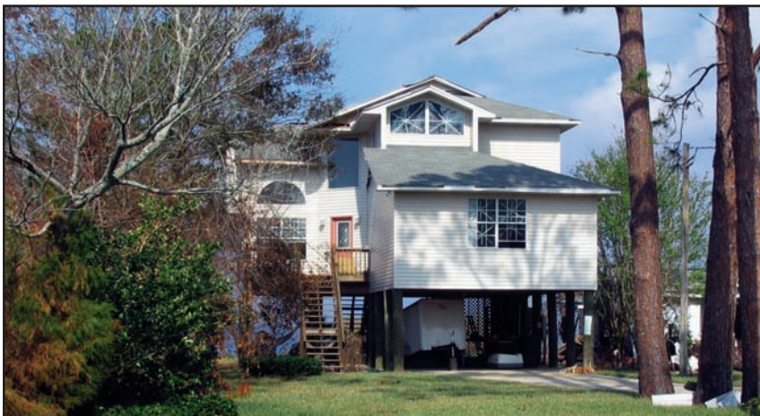
Figure 5-10. BIG LAGOON, FLORIDA: This house was elevated on piles, preventing severe damage from coastal flooding. (Source: FEMA 489)
