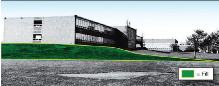
Figure 5-22: High school in Bloomsburg, PA, elevated on fill
