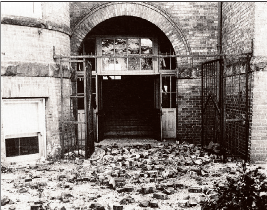
Figure 4-20: Another dangerous entry collapse, Seattle, WA, 1949
