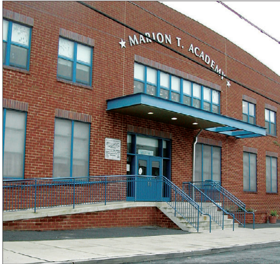
Figure 5-23: A stemwall foundation elevates the Marion T. Academy above the flood level in Wilmington, DE.
