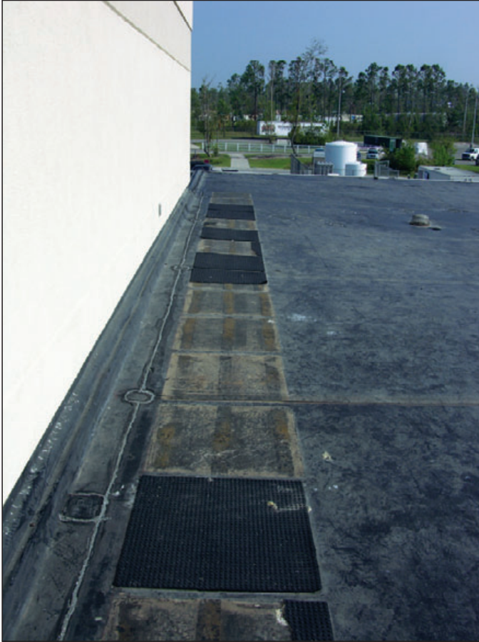
Figure 6-87: Several rubber walkway pads were blown off the single-ply membrane roof. Estimated wind speed: 130 mph. Hurricane Katrina (Mississippi, 2005)
