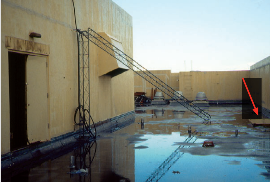
Figure 6-139: The antenna collapsed and was whipped back and forth across the roof membrane. Hurricane Andrew (Florida, 1992)
