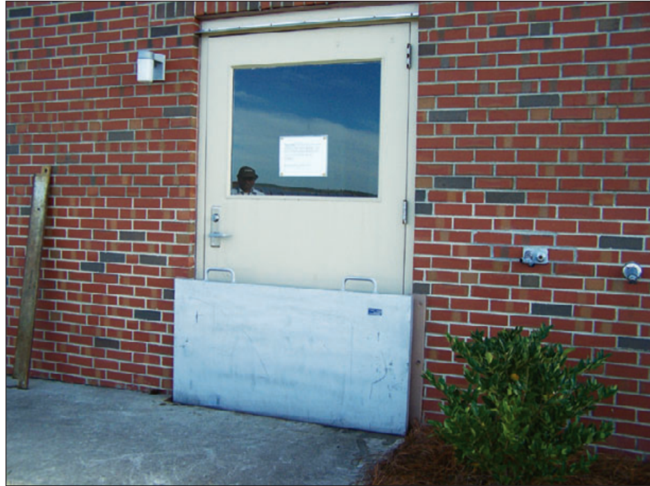
Figure 5-26: Specially designed panels are mounted to block doors, windows, and other openings to keep water from entering the building.
