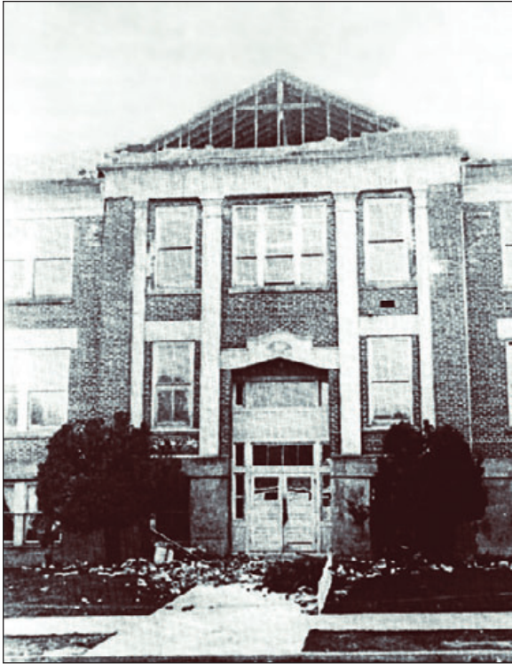
Figure 4-19: The student body president was killed here by falling brickwork, Seattle, WA, 1949
