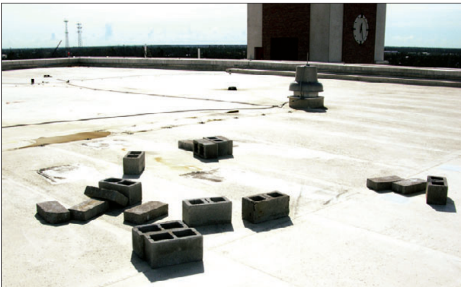
Figure 6-108: A satellite dish anchored similarly to that shown in Figure 6-107 was blown off this five-story building. Estimated wind speed: 140–160 mph. Hurricane Charley (Florida, 2004)
