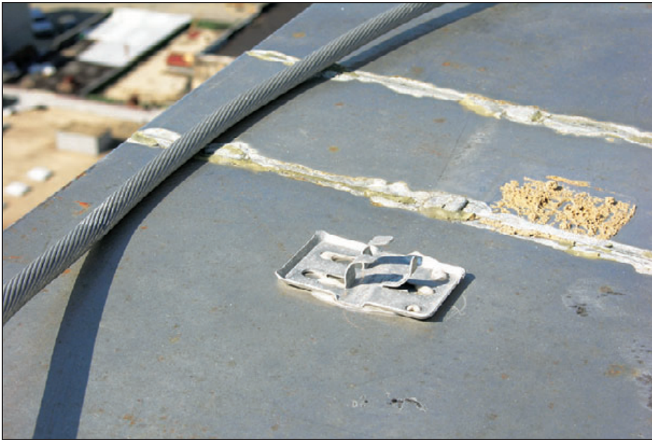
Figure 6-111: This conductor connector was adhered to the coping. The conductor deformed the connector prongs under wind pressure, and pulled away from the connector. Estimated wind speed: 130 mph. Hurricane Katrina (Mississippi, 2005)
