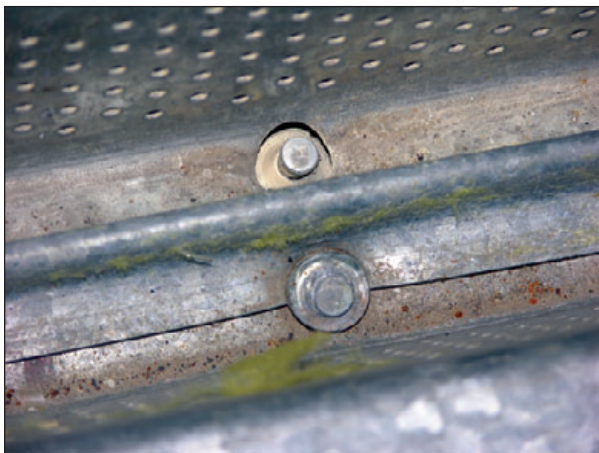
Figure 6-37: Looking down at a sidelap of a deck attached with powder-driven pins. The washer at the top pin blew through the deck.
