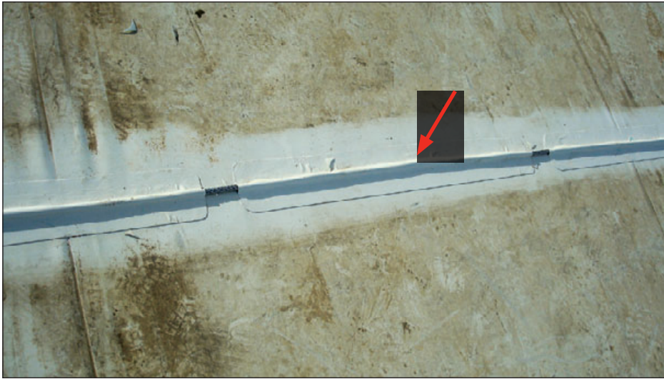
Figure 6-114: Use of intermittent membrane flashing strips to secure an LPS conductor, as illustrated in Figure 6-113
