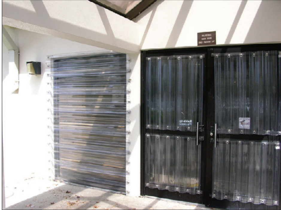
Figure 6-127: Polycarbonate shutters were temporary screwed to the doors and wall adjacent to the window opening. An advantage of polycarbonate is its translucence, which allows daylight to enter the building without removing the shutters. Hurricane Francis (Florida, 2004)
