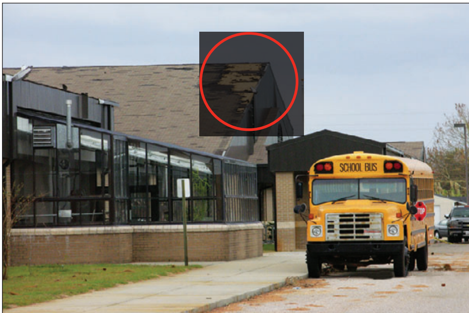
Figure 6-12: Constructed in 1995, this school was used as a hurricane shelter. The large number of occupants moved from one area of the school to another as water entered various areas of the building due to envelope failures. Estimated wind speed: 105 to 115 mph. Hurricane Ivan (Florida, 2004)
