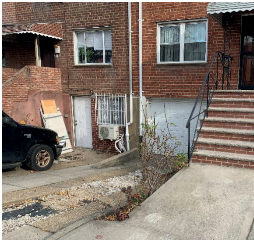
c. Driveway sloping down to converted basement
