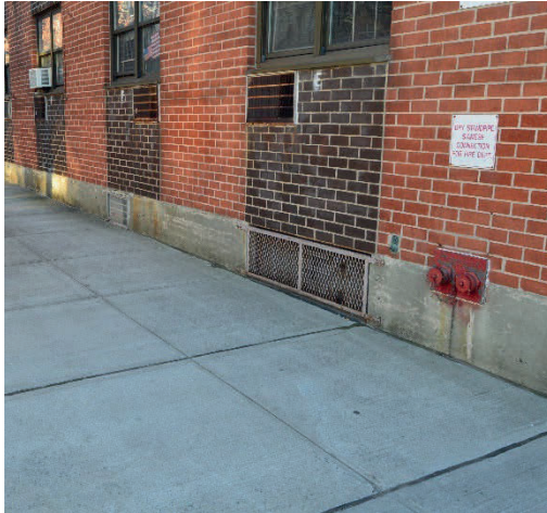
a. Ventilation openings near sidewalk level
