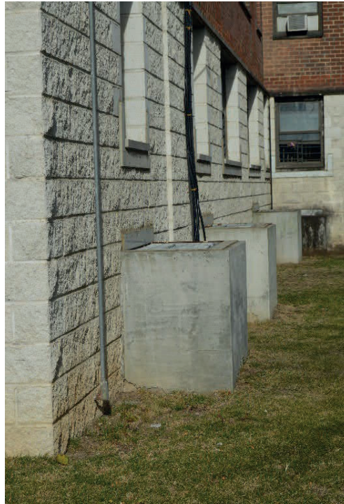
Figure 12. Vents retrofit by extending vent wells above ground level
