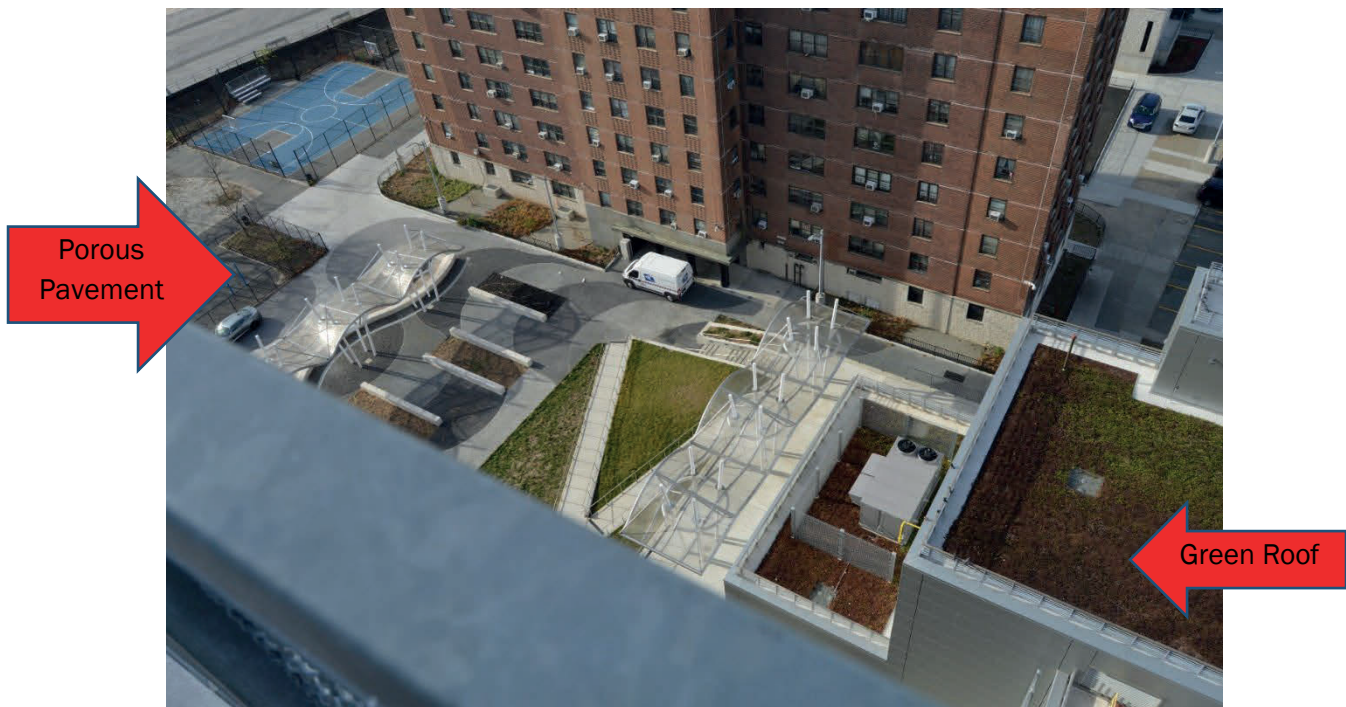
Figure 5. New York City site with porous pavement and green roof
