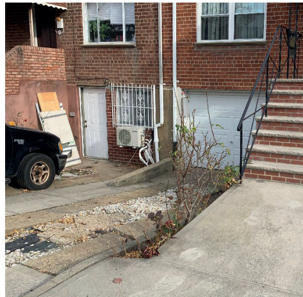
Figure 5. Basement window too high and too small for escape (left) and basement window with security bars (right)
