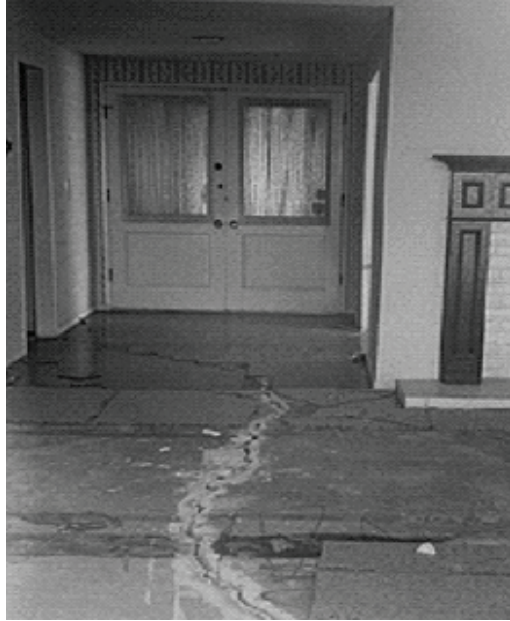
Figure 4-12 Example of damage caused in building on cut and fill site. The line of slab damage follows the transition from cut soils to fill soils.
