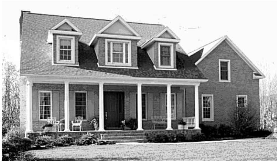
Figure 6-12 House constructed with masonry walls.
