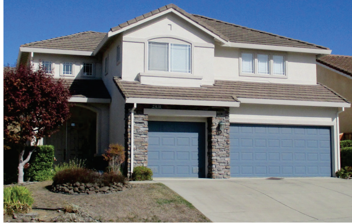
Figure 11-9 A common living-space-over-garage dwelling.
