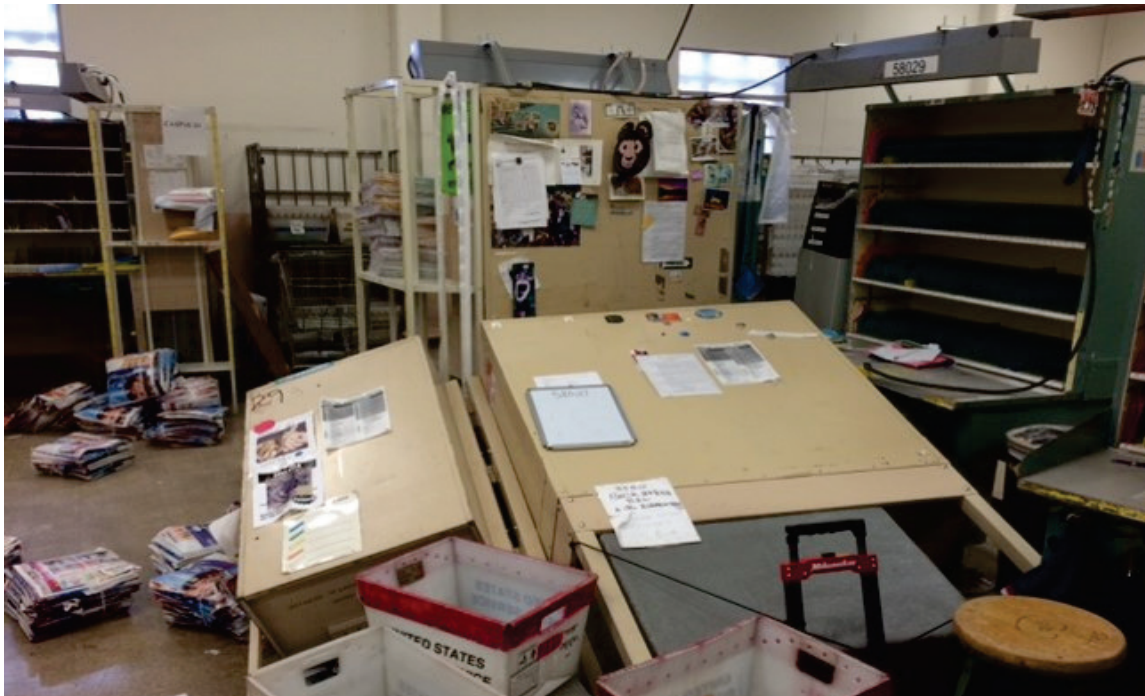
Figure 10-3 Toppling of unanchored cabinets in the 2014 South Napa Earthquake (from Glen Granholm, EERI Learning From Earthquakes).
