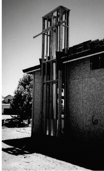
Figure 9-6 Factory-built flue and light-frame enclosure.
