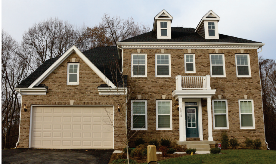
Figure 7-2 Dwelling with masonry veneer.
