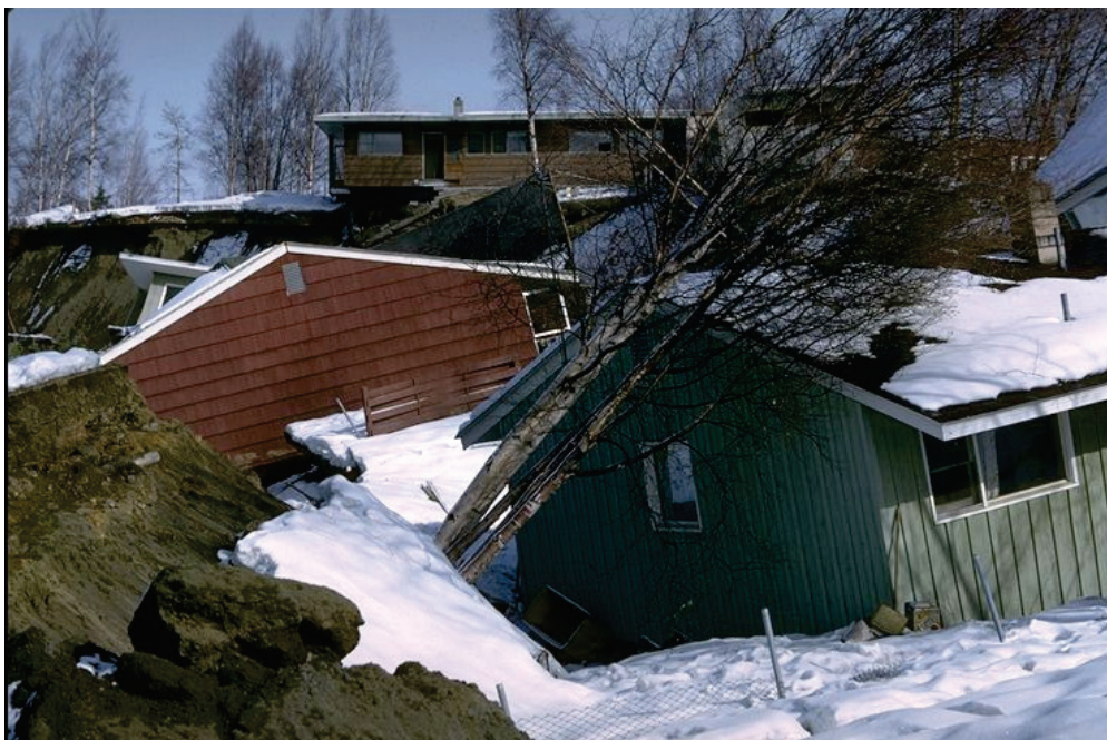
Figure 2-6 Dwellings damaged due to a landslide at the site during 1964 Anchorage Earthquake (from National Information Service for Earthquake Engineering, NISEE).
