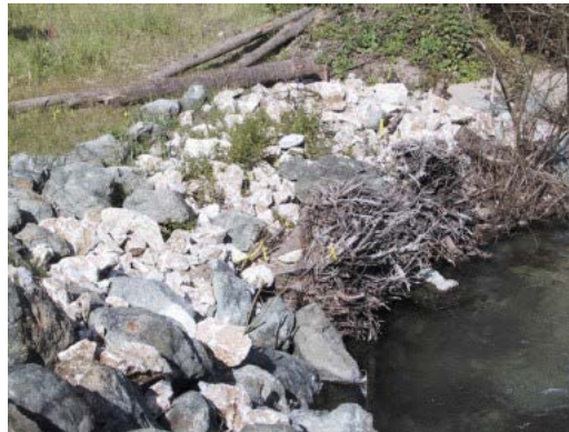
Figure 5.1.8. Nature-based solutions or hybrid approaches to streambank stabilization (combining hardscapes with nature-based solutions) can protect trails and other park facilities.
