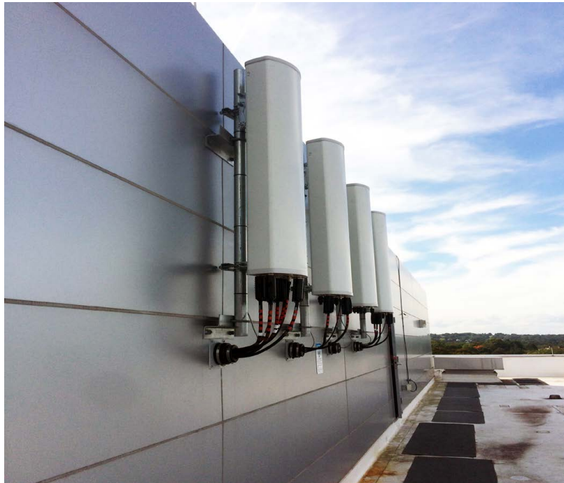
Figure 4.4.3. Antennas can be secured to the building structure to improve wind resistance.
