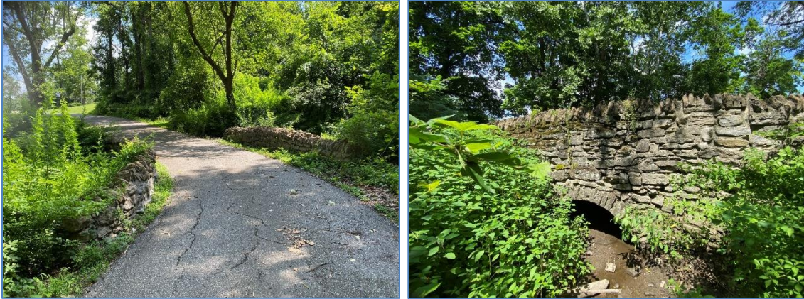
Winding drives with a view of the contributing stone bridge in Putnam Hill Park.
