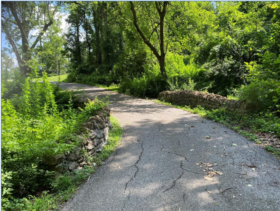
Figure 6: Stone bridge associated with Putnam Hill Park drive. Applicant photo.
