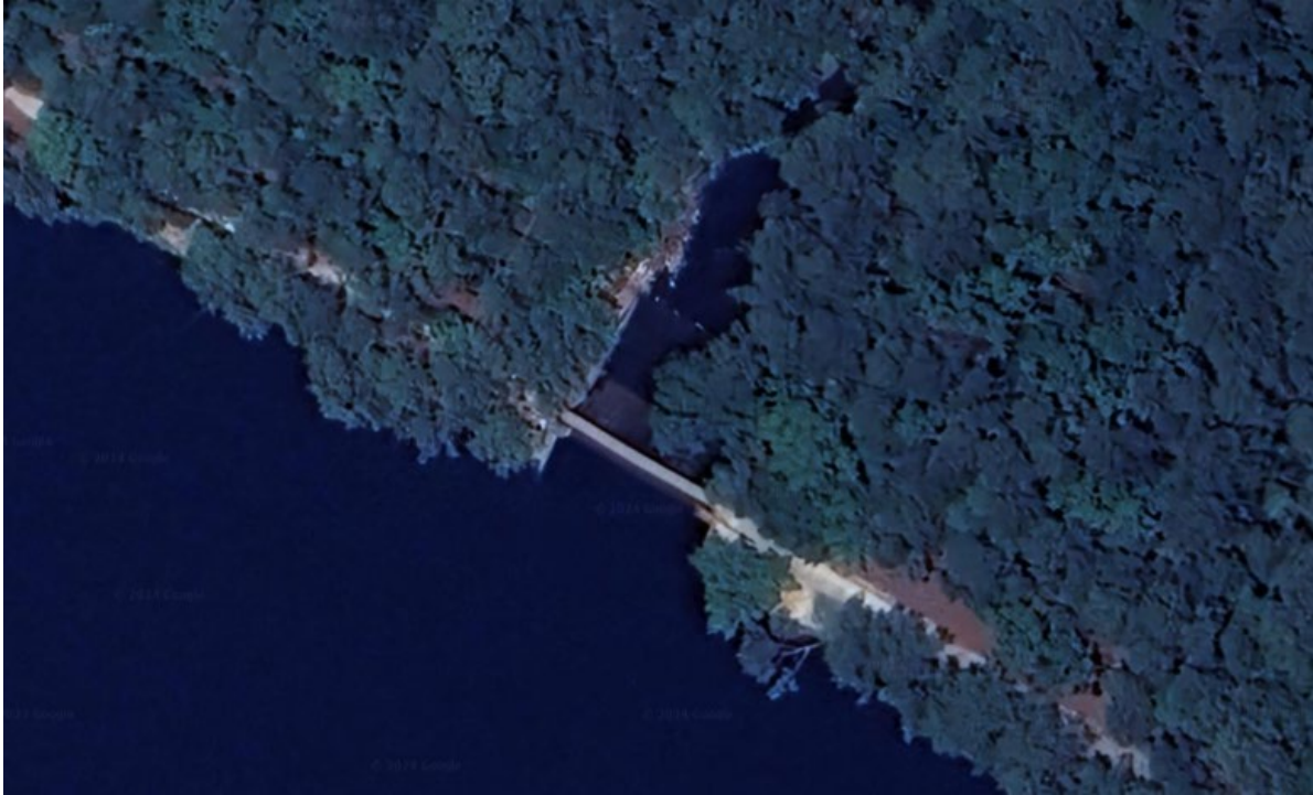
Figure 7. Aerial Image from Google Earth of a Dam Emergency Spillway
