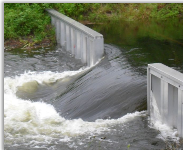
Figure 22. Weir Abutment Perpendicular to flow
