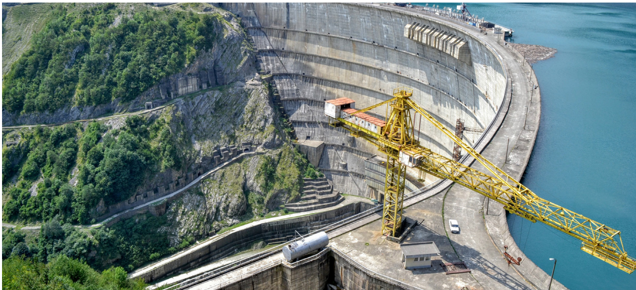
Dam Under Construction, Source: Alex Bagirov
