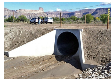
To prevent flooding and erosion this culvert was replaced with a larger culvert and additional wingwalls.
