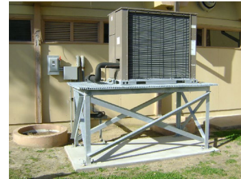
An elevated heat pump is an example of elevating equipment to prevent flooding damage.
