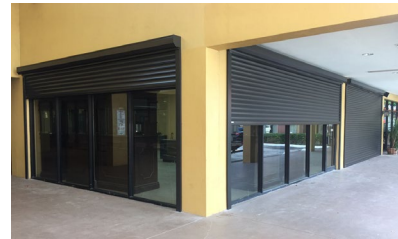
Adding hurricane shutters protects windows against flying debris during high wind events such as hurricanes, tropical storms, or severe storms.
