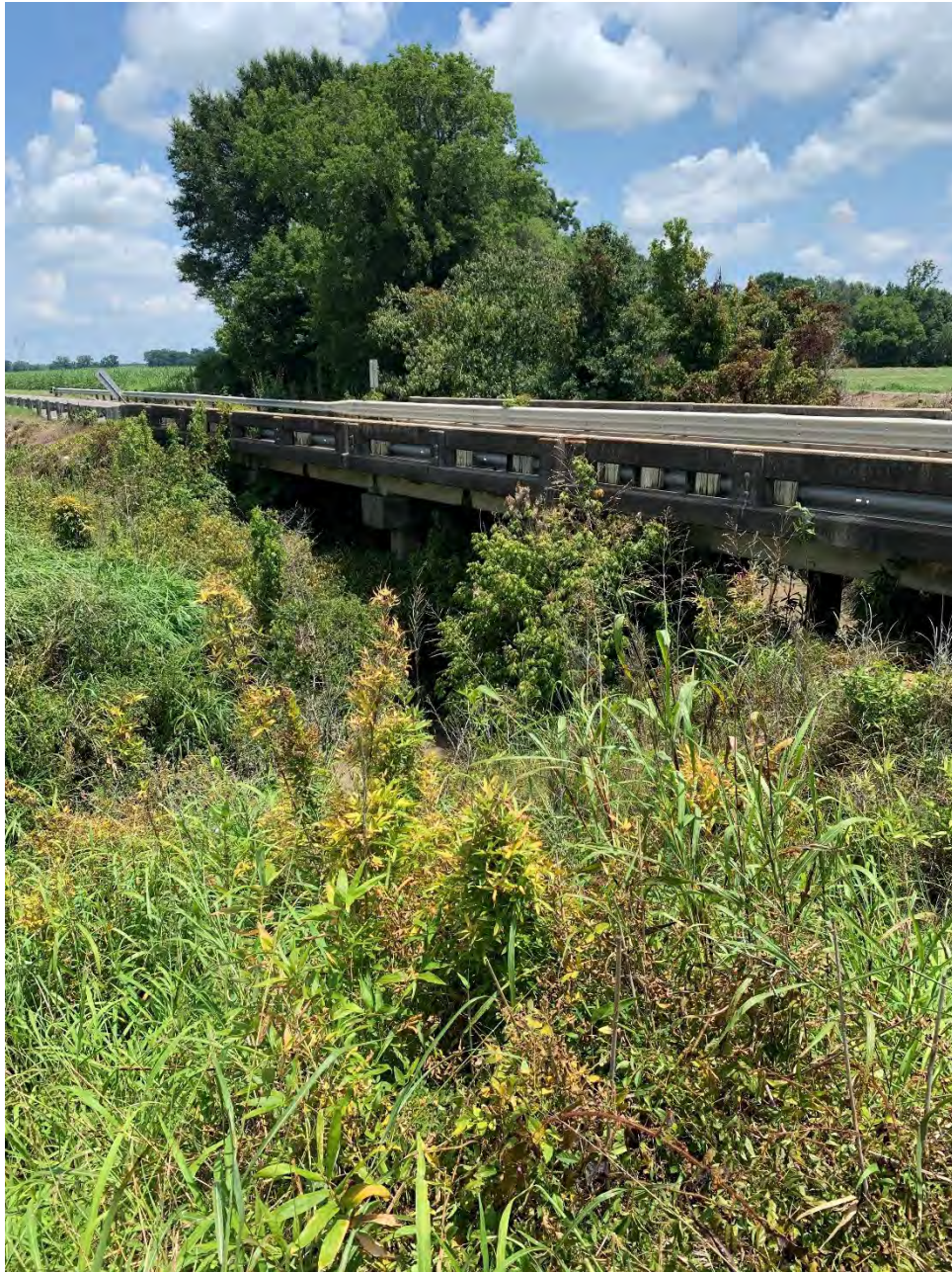
Figure 8. West detail of the bridge at the LA Hwy 984 (Rougon Road) crossing where slope stabilization measures will be applied.
