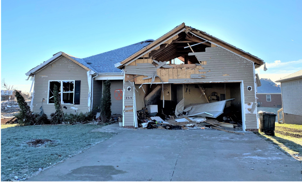
Figure 7. Loss of roof sections and gable end framing initiated from garage door failure Bowling Green, Kentucky (December 2021)
