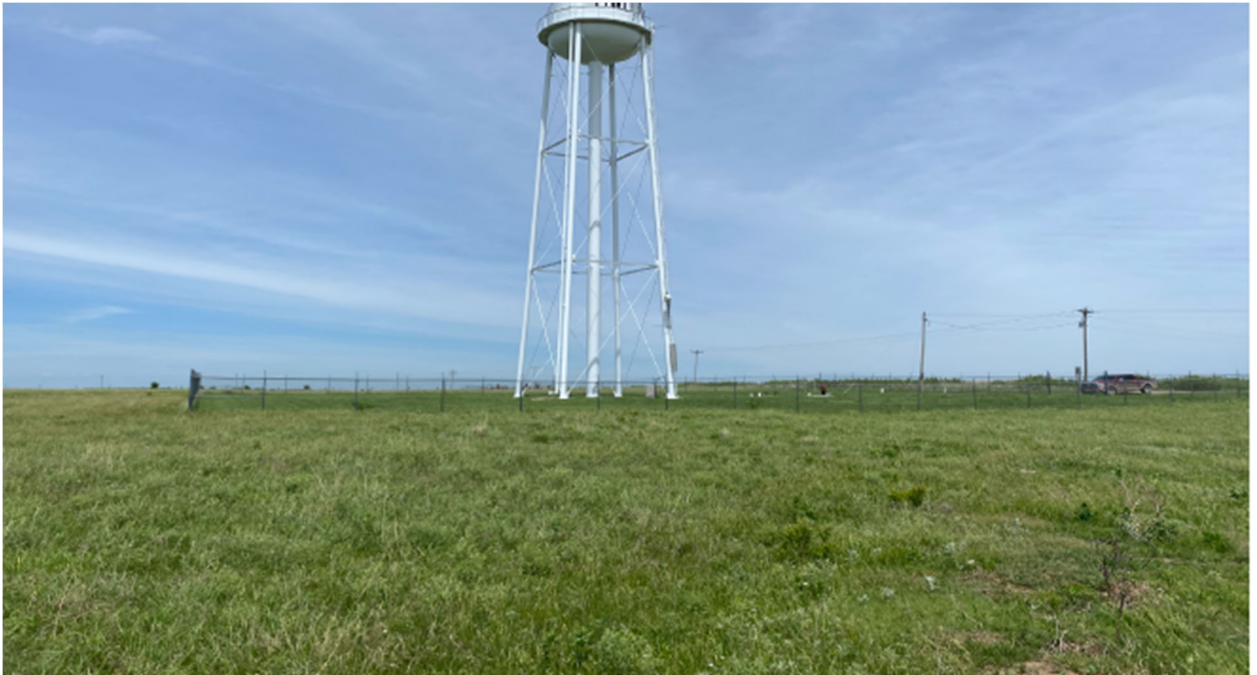
Figure 13: View from the substation location looking North/Northeast toward the K-57 Highway
