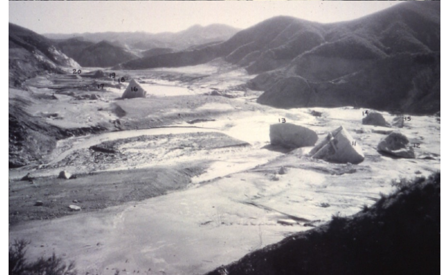
St. Francis Dam, CA 1928
