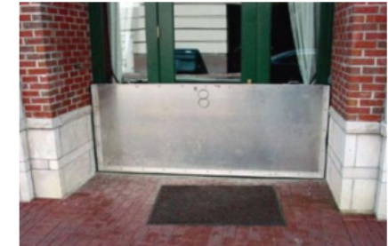
Figure 1. Photo showing an example of a floodgate to keep floodwaters out of a building entrance.
