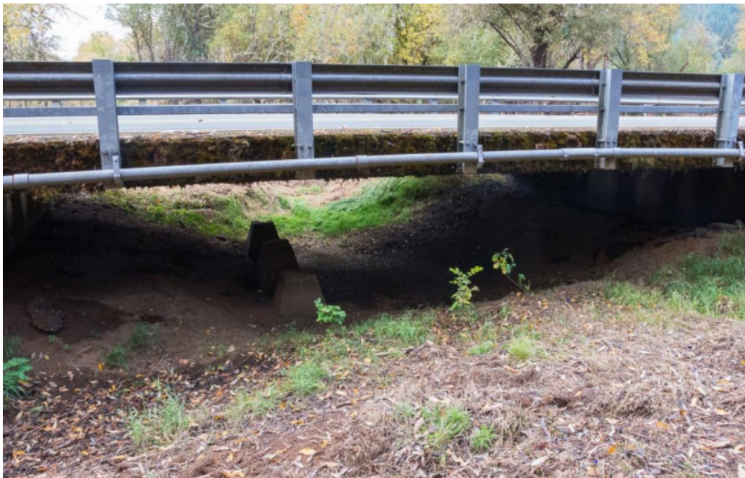
Figure 4: View of existing south bridge (04057B)
