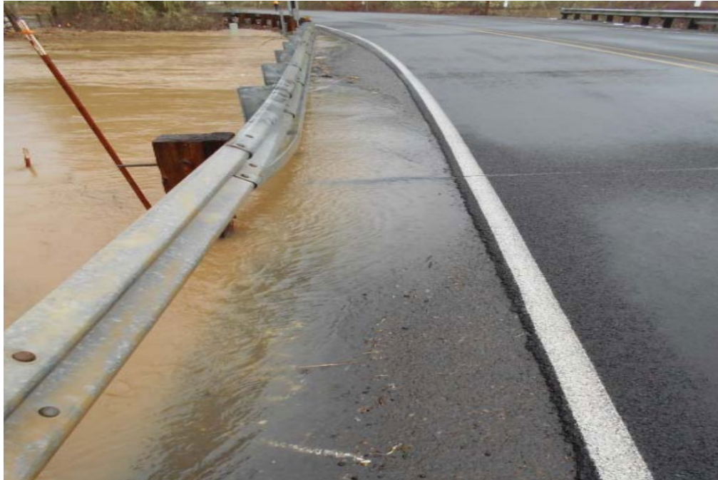
Figure 7: Flooding along the western roadway shoulder at north bridge (04057A) resulting in the erosion of the roadway shoulder
