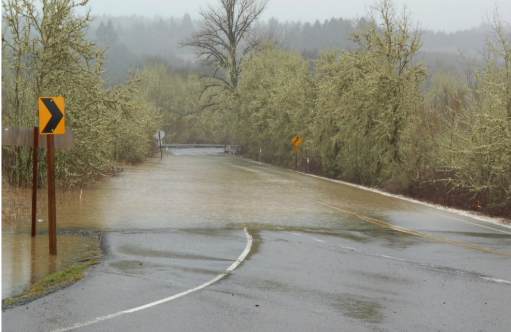
Figure 6: Example of substantial flooding at the intersection of Territorial Highway and Lorane Highway from February 2014
