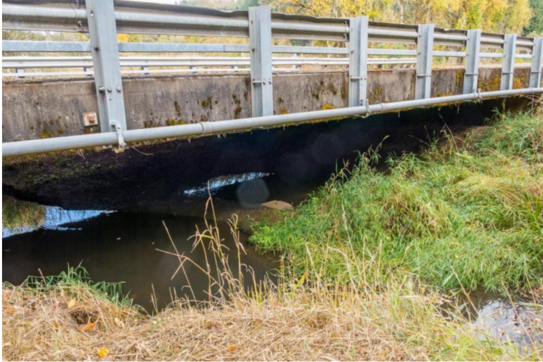
Figure 3: View of existing north bridge (04057A)
