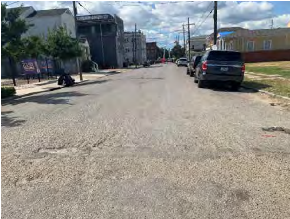
Figure 18: Typical conditions of Baronne Street, as seen from its intersection with Martin Luther King Jr. Boulevard, where the road reconstruction with bioswales is proposed
