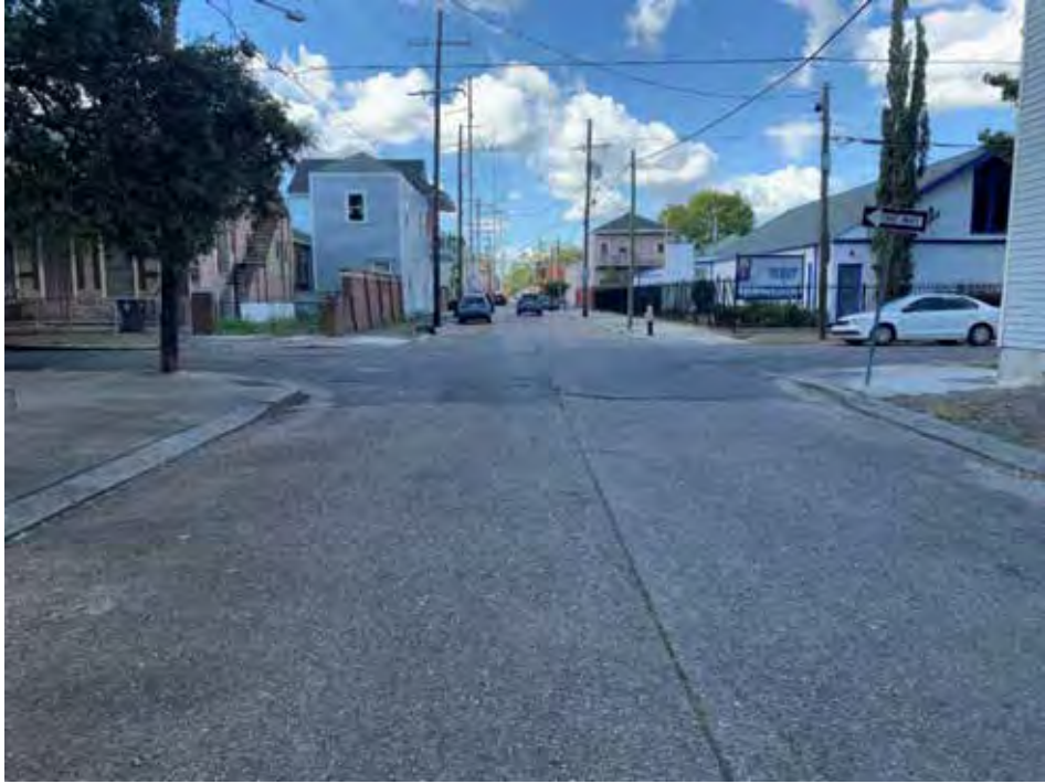
Figure 15: Typical conditions of Annunciation Street, as seen from its intersection with 3 rd Street
