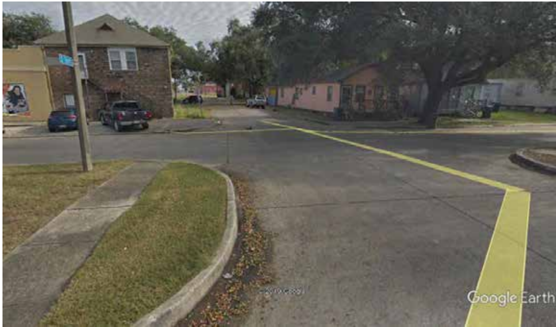
Figure 8. Representative view of Tonti St. (Google Street View, 11/2018), looking northeast from Toledano St. Scope of work along six blocks of Tonti St. from Toledano to Martin Luther King Jr. Blvd. includes replacement of roadway, construction of ADA ramps at street corners, replacement of sidewalks, and replacement of existing drainage pipes and structures with green infrastructure drainage design in the area between the roadway and edge of right-of-way. This area is not within an a NRHP listed/eligible historic district.
