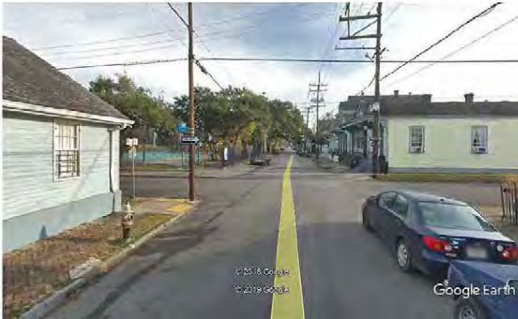
Figure 22. View of intersection at Chippewa and Third St. (Google Street View, 12/2018), looking northeast. Scope of work entails replacement of water lines; construction of a green intersection at this location, including replacement of roadway, construction of green drainage system under roadway, installation of permeable paver crosswalks and gutters, construction of vegetated street basins, narrowing of the roadway; and construction of ADA ramps and replacement of curbs and sidewalk. This area is located within the NRHP listed Irish Channel Historic District.
