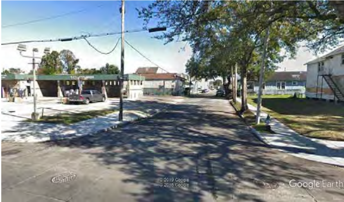
Figure 19. Representative view of Dryades St. (Google Street View, 11/2018), looking northeast from Louisiana Ave. Scope of work along ten blocks from Louisiana Ave. to Philip St. includes construction of ADA ramps at street corners, and replacement of roadway curbs, and existing water and drainage pipes and structures within the existing right-of-way. This area is located within the NRHP listed Central City Historic District.
