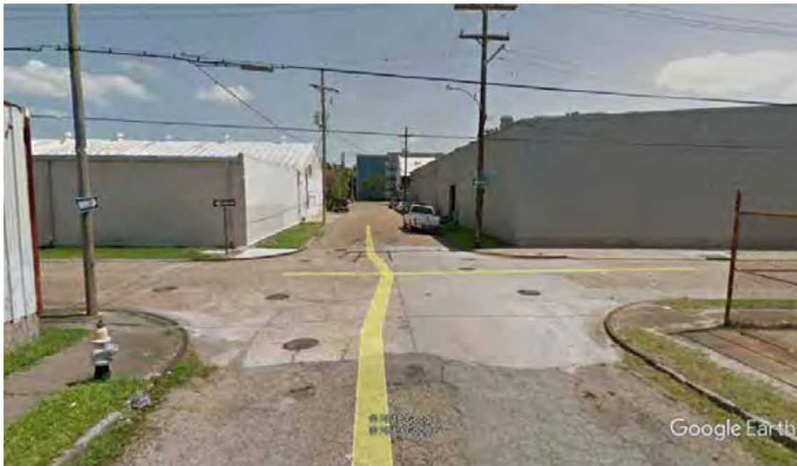
Figure 18. View of intersection at St. Thomas St. and Orange St. (Google Street View, 11/2018), looking northeast. Scope of work entails construction of a green intersection at this location, including replacement of roadway, construction of green drainage system under roadway, installation of permeable paver crosswalks and gutters, and construction of ADA ramps and replacement of curbs. This area is located within the NRHP listed Lower Garden Historic District.
