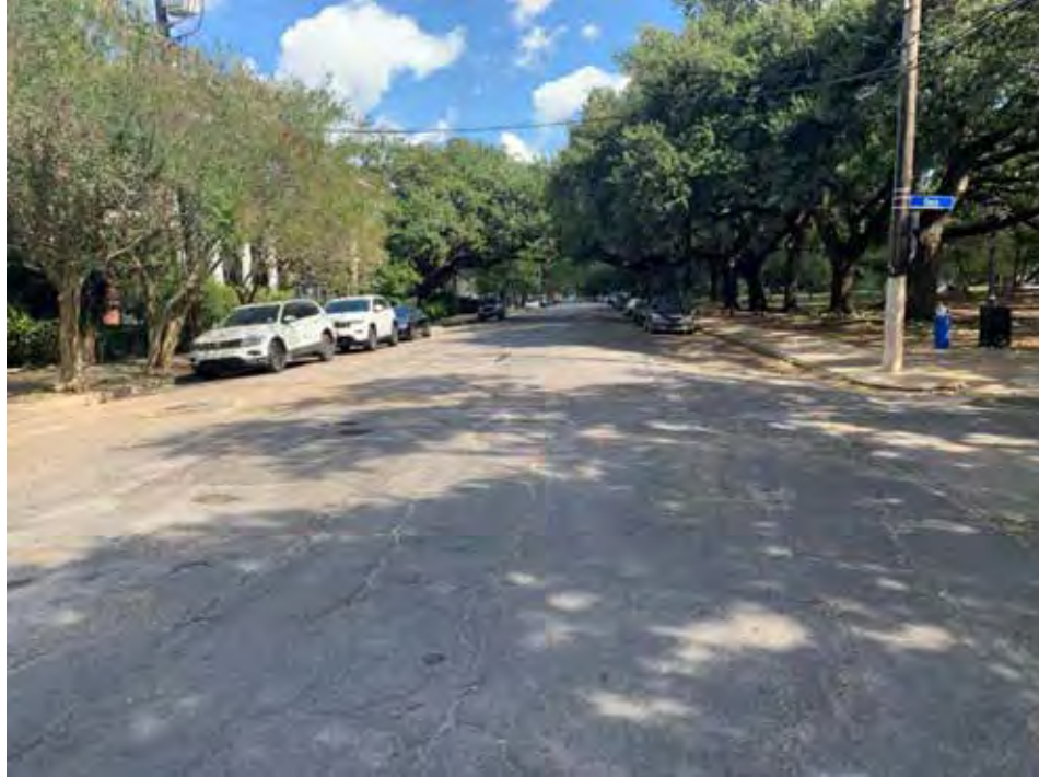
Figure 23: Typical conditions of Coliseum Street as seen from its intersection with Race Street, where the road reconstruction with bioswales is proposed
