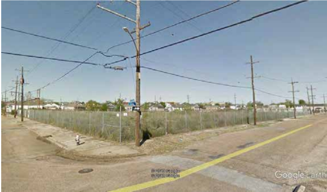
Figure 26. View of Saratoga Square, looking west (Google Earth Street View, 11/2018). Scope of work includes demolition/replacement of sidewalks, curbs, ADA ramps, and small segments of roadway around the perimeter of the city block; demolition/clearing of block; excavation and construction of multiple, interconnected detention ponds for the collection of stormwater; construction of supporting surface and underground drainage structures, interior park sidewalks; and planting of trees, shrubs, and groundcover. This area is located within the NRHP listed Central City Historic District.
