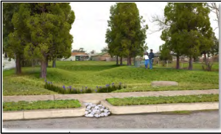
Photograph 1. An example of a completed stormwater lot
