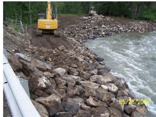
USACE emergency riprap section, northwest of bridge.
