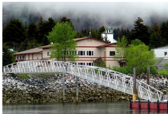
Ferry Dock Refurbishment
