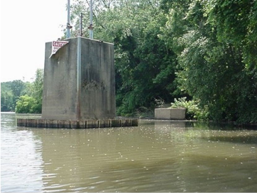
Figure 2: Existing intake structures are no longer easily accessible, and sediment has built up around the structures.
