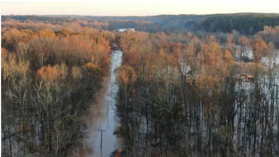
Figure 4: The access road to the pump station is completely submerged for several thousand feet during flood events.
