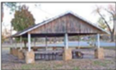
Picnic shelter / east
