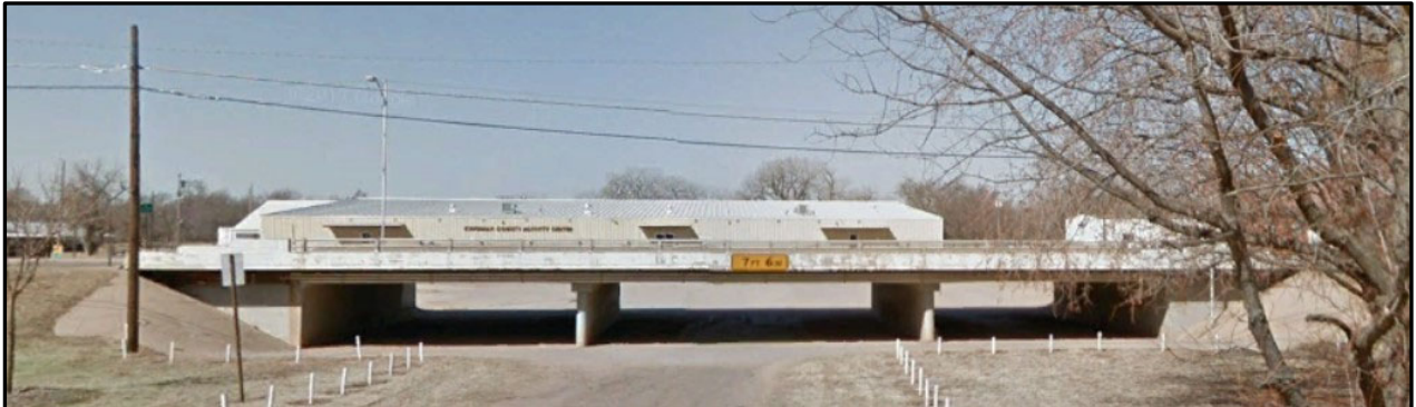
Main Street underpass, view to west Source: Google Earth street view (Imagery date – February 2022)
