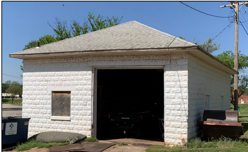
Storage Building ca. 1925 view to west
