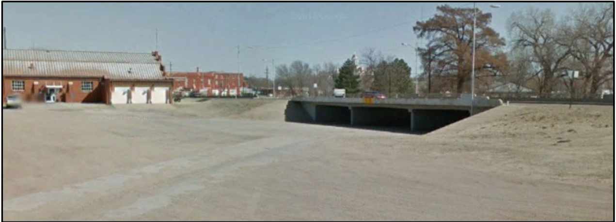
Main Street underpass, view to northeast Source: Google Earth street view (Imagery date – February 2022)
