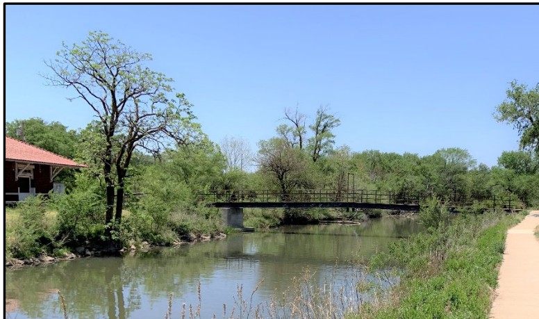
Foot bridge over mill race – view to west (note concrete walking path at right of photograph and Missouri Pacific Railroad depot at left of photograph)
