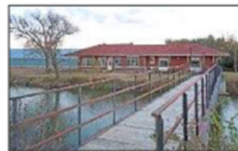
Pedestrian bridge over mill race
