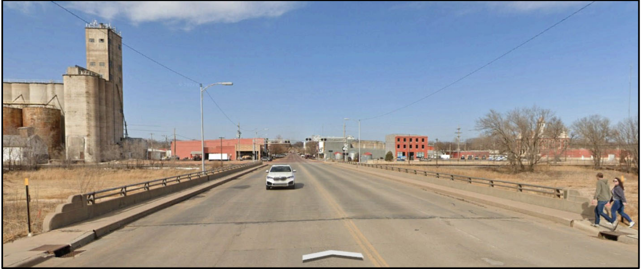
Main Street crossing S Fork Ninnescah River, view to north Source: Google Earth street view (Imagery date – February 2022)
