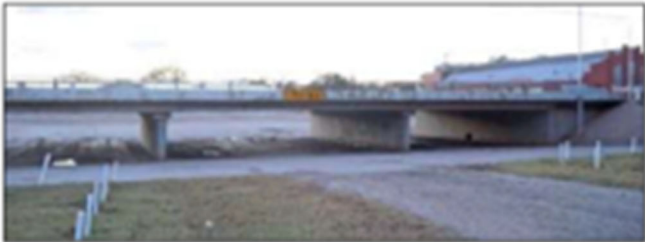
Main Street underpass (view from Riverside Park)
