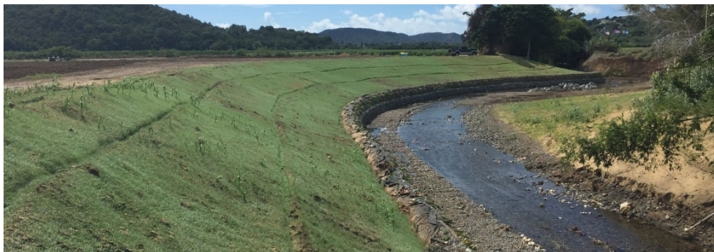
Figure 3-1: Hydroseeding along the Río Loco channel banks. (Photo credit: PDC)
