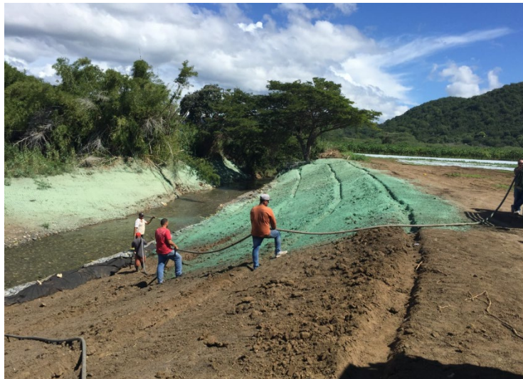
Figure 2-1: Hydroseeding performed by Protectores de Cuencas to help restore the banks of the Rio Loco in Yauco (Photo credit: PDC)
