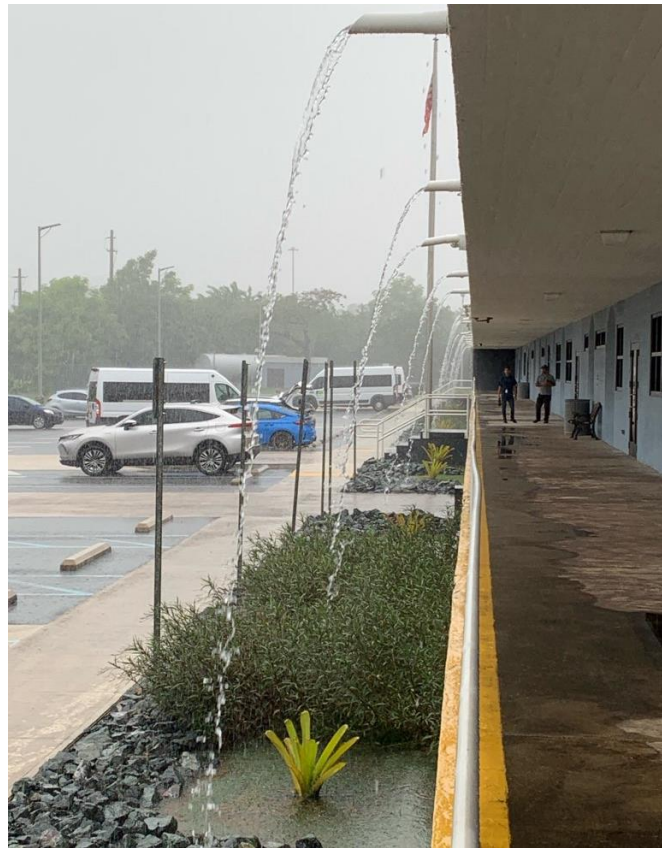
Figure 2-4. Bioretention planter boxes at the GSA federal facility in the municipality of Guaynabo during an afternoon rain
