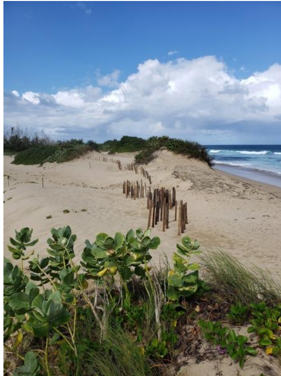
Figure 0-16: Sand-trapping devices used by Vida Marina (NOAA)
