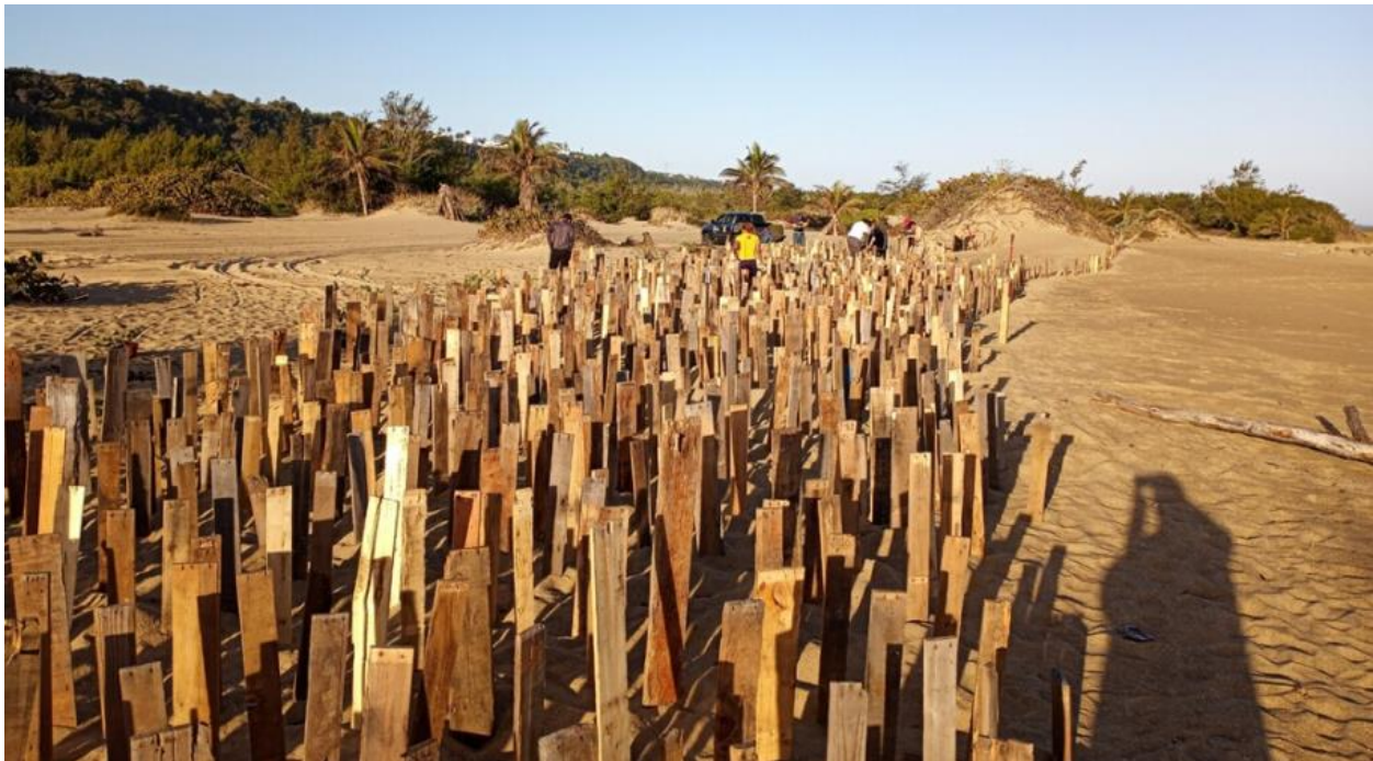
Figure 0-13: Sand matrix typical layout (R.J. Mayer, used with permission)
