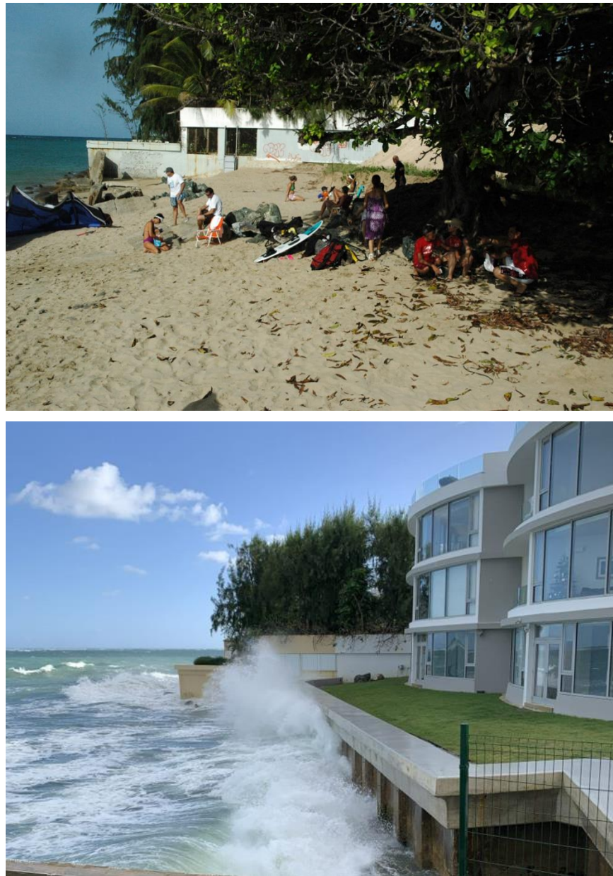
Figure 0-2: Top: former sandy beach at Punta Las Marías in San Juan, Puerto Rico. Bottom: same site after the construction of a steel sheet pile bulkhead with a concrete cap to manage swells and coastal flooding. The bulkhead exacerbated the loss of sand, further coastal erosion at the toe of the structure, reduced public access and the loss of recreational and ecological values once associated with this beach area (N. Pérez, used with permission).
