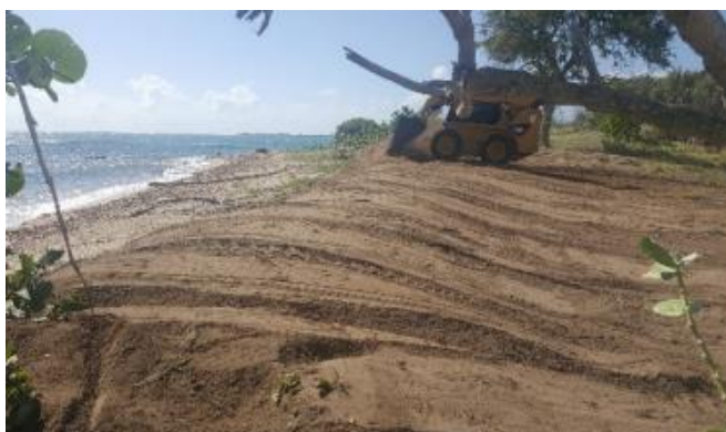
Figure 0-18: Construction of sand mounds at Playa Tamarindo (Protectores de Cuencas, used with permission)
