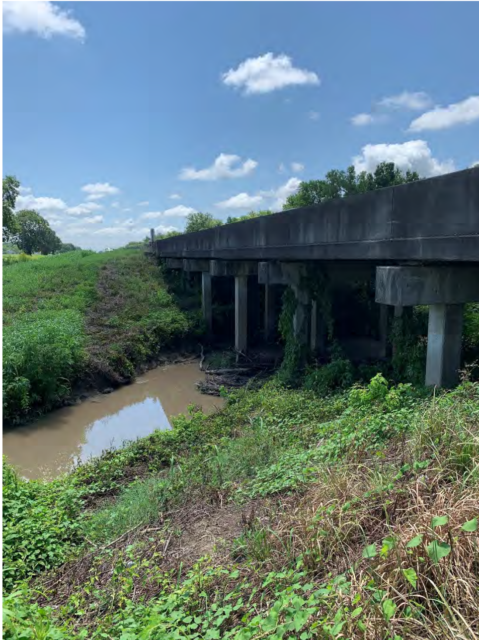
Figure 10. North detail of the bridge at the US Hwy 190 crossing where slope stabilization measures will be applied.
