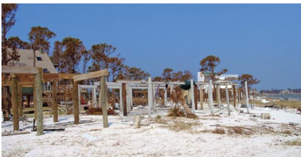
Several structures were completely torn off their pile foundations during Hurricane Ivan as a result of significant flood depths, waterborne debris impacts, and lack of connections.
