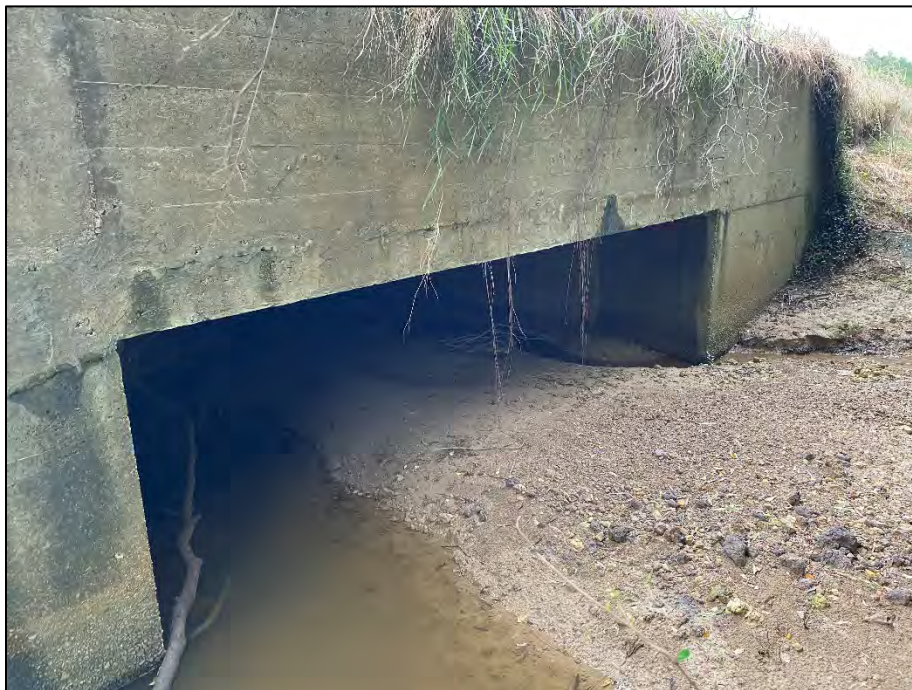
PHOTO 4 Existing Culvert Under BI Canal
