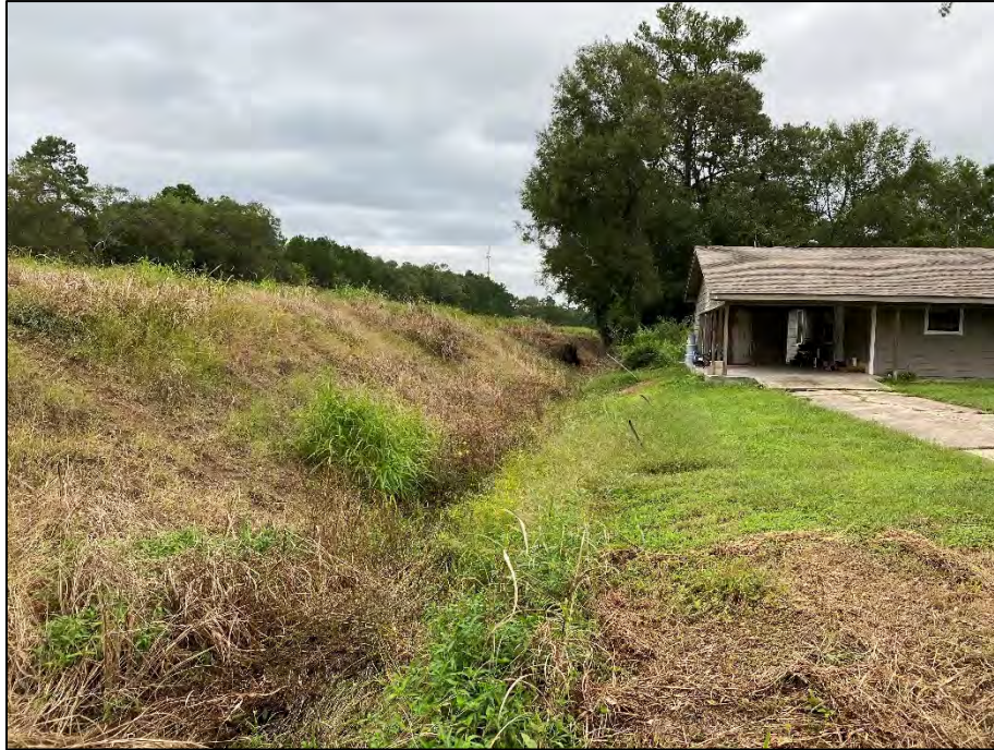
PHOTO 3 Existing Weep Ditch Along East Side of BI Canal
