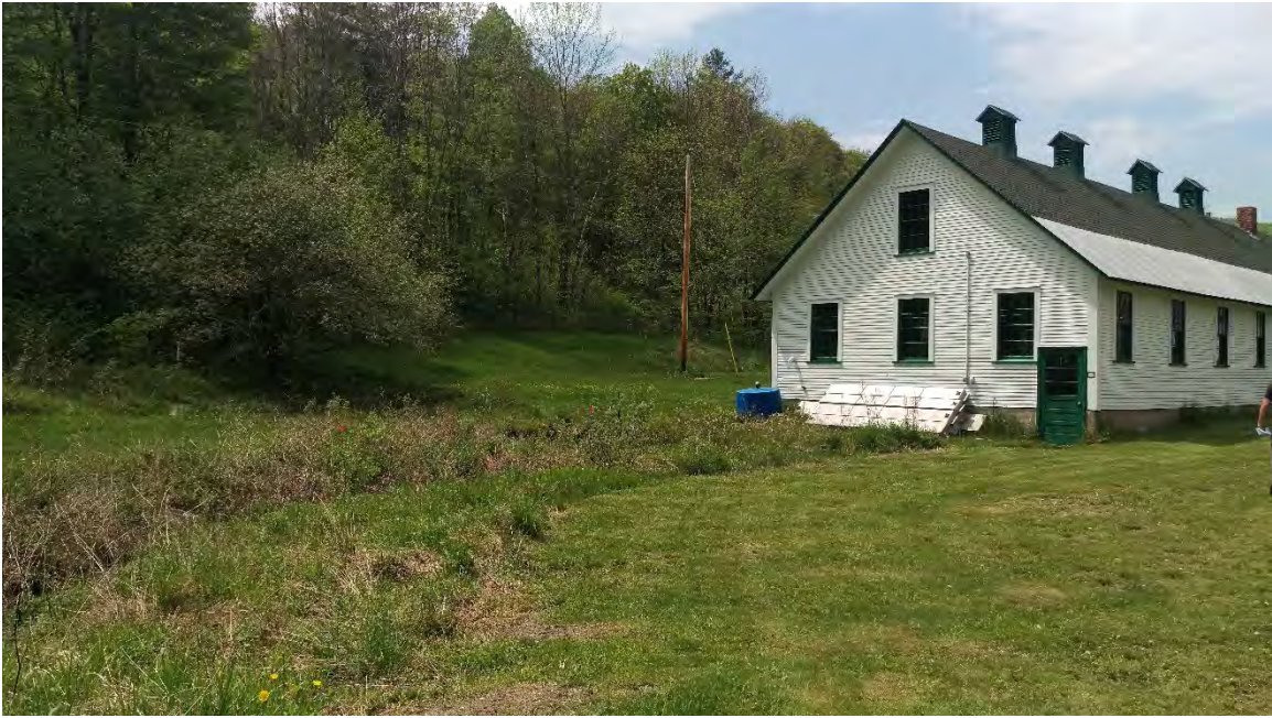
Photograph 5: Hatchery Building, looking north.
