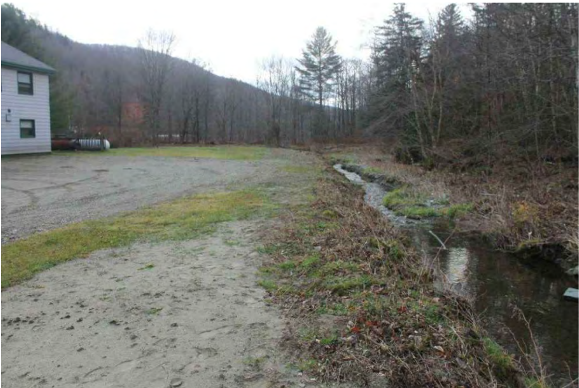
Photograph 12: Area south of the dam, looking south.
