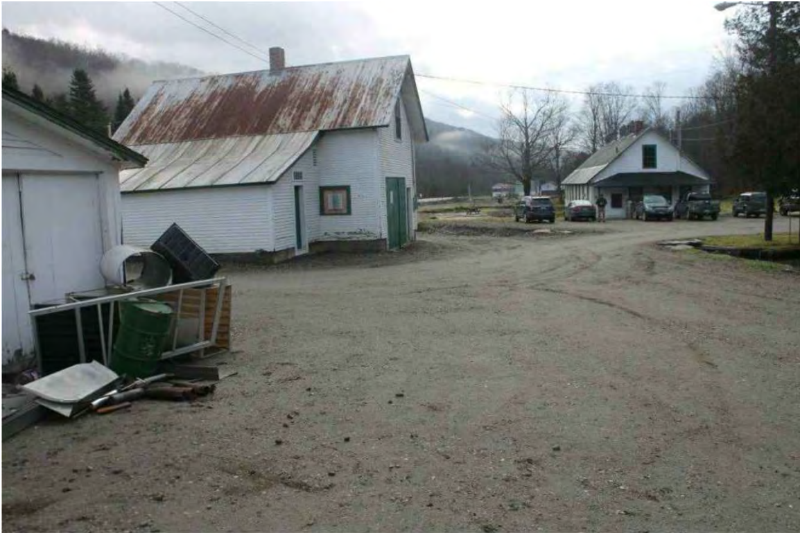
Photograph 3: Garage and Freezer House, looking south.
