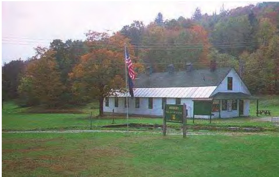
The Hatch House shortly before Tropical Storm Irene, looking southwest.
