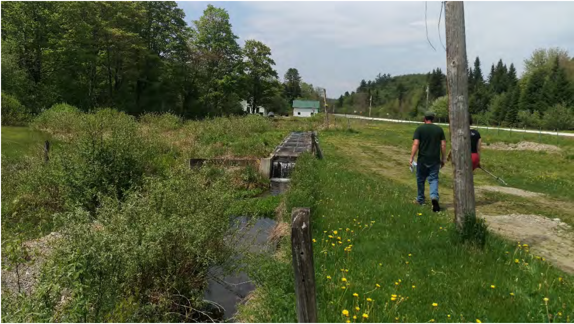
Photograph 9: Concrete raceway (center) flowing into Pond #5 (lower left), looking north.
