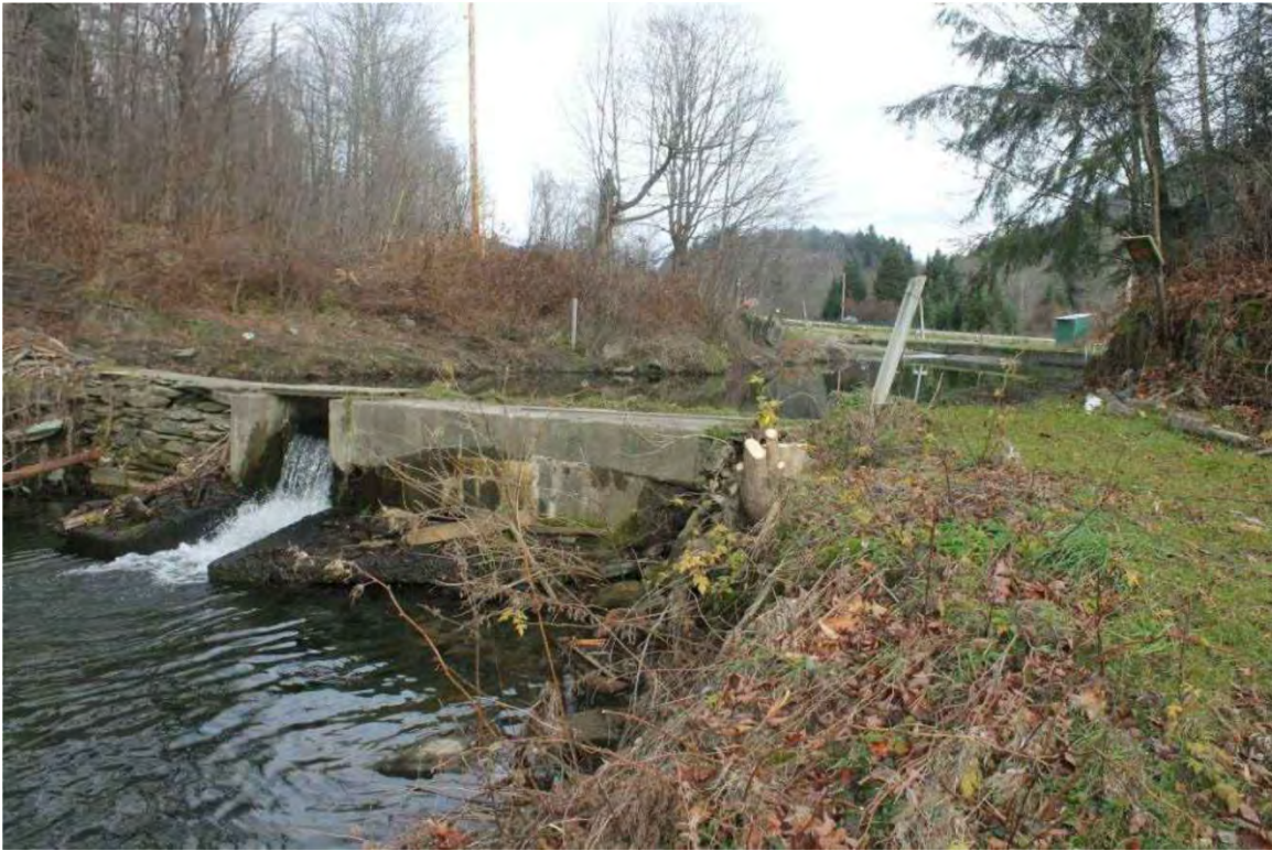
Photograph 11: Dam at south end of Pond #5, looking north.
