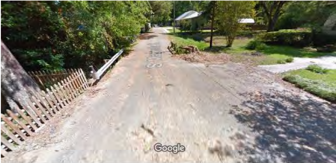
Figure 14 – Street view of the South Magnolia Street Bridge (Image Source: Google Maps)
