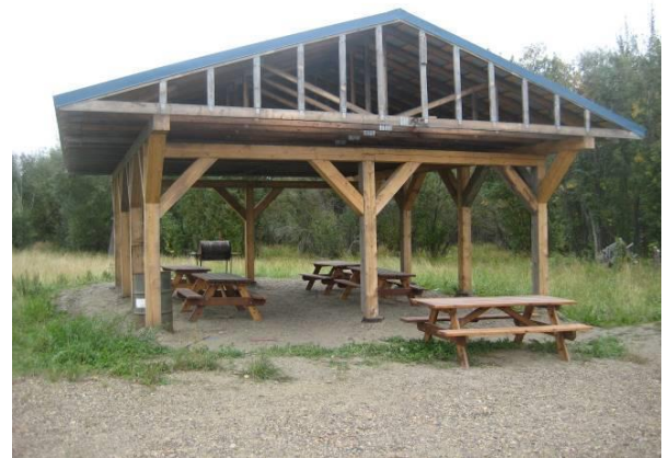
Figure 4. The finished picnic pavilion at the ball field site.
