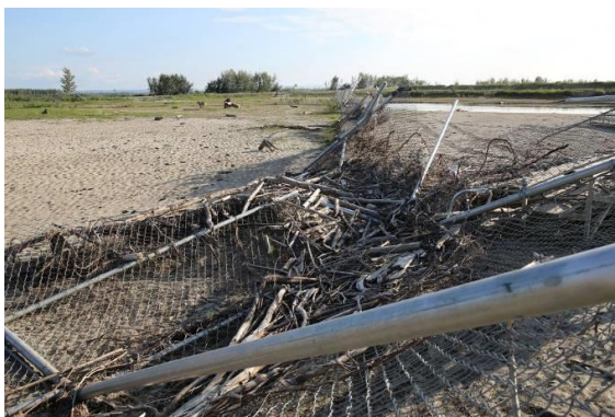
Figure 2. The fence running along the Galena ball field sits ruined after the floodwaters receded.
